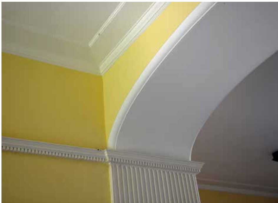
40. Architectural details from c.1905 from the passage side of the archway into the stairhall.
