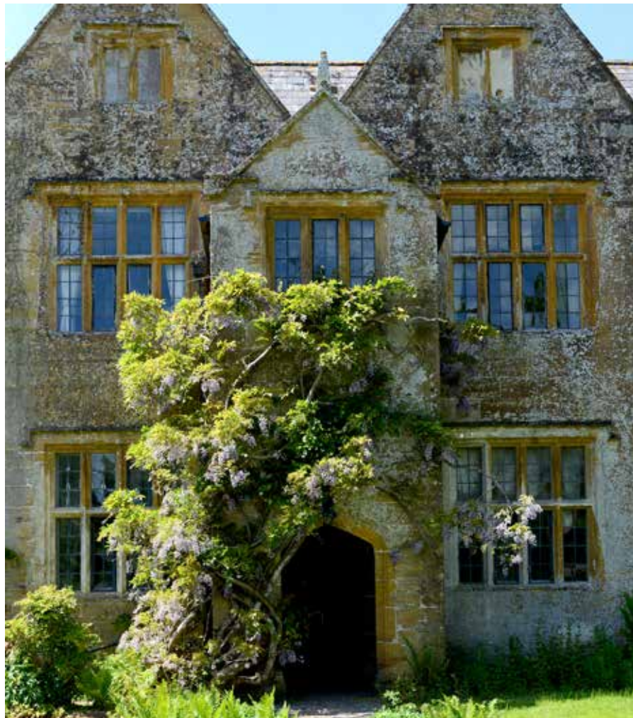
8. The porch in the middle of the east front.
