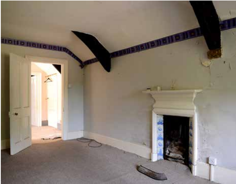
29. The arch braces of the southern two trusses looking northeast.
