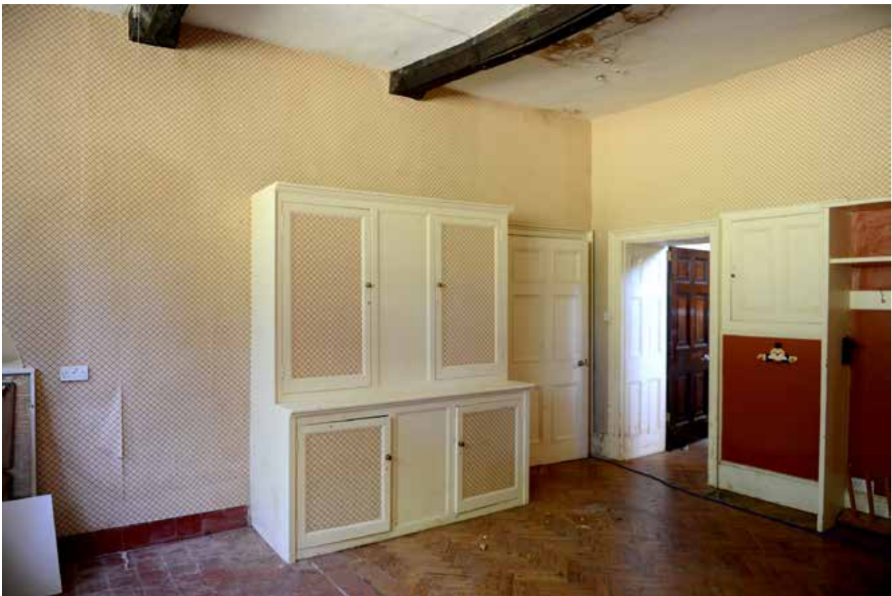
31. The service room looking southeast.
