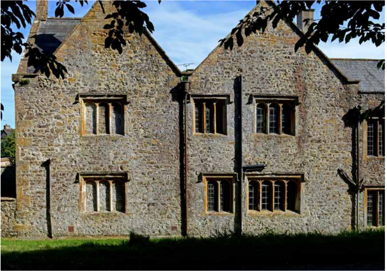
25. The north front of the main block.
