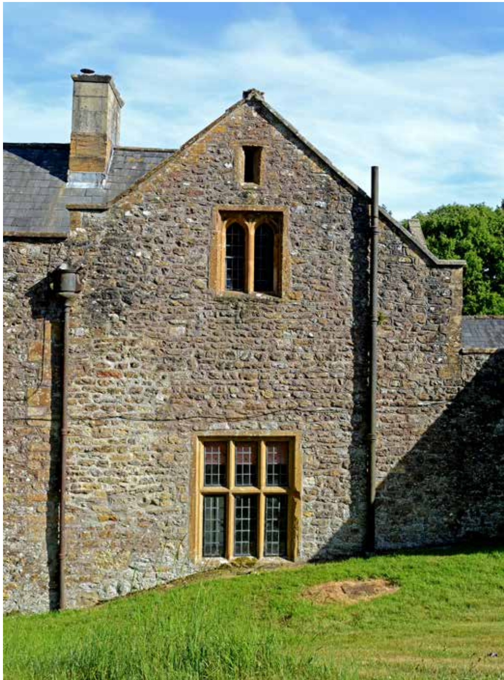
27. The north end of the west range.
