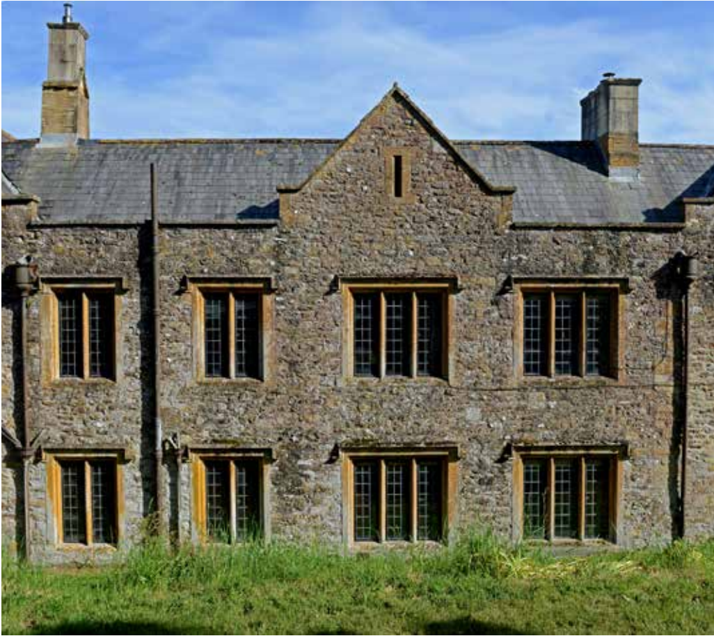
26. The north front of the link block.
