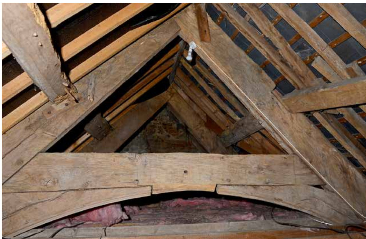
28. The upper part of the second truss from the south end.
