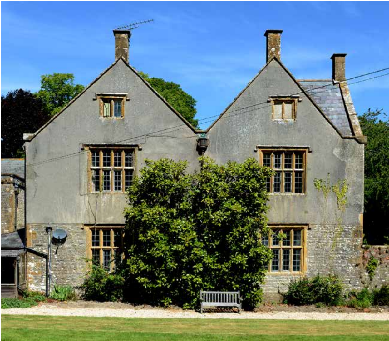
12. The south front of the main block.
