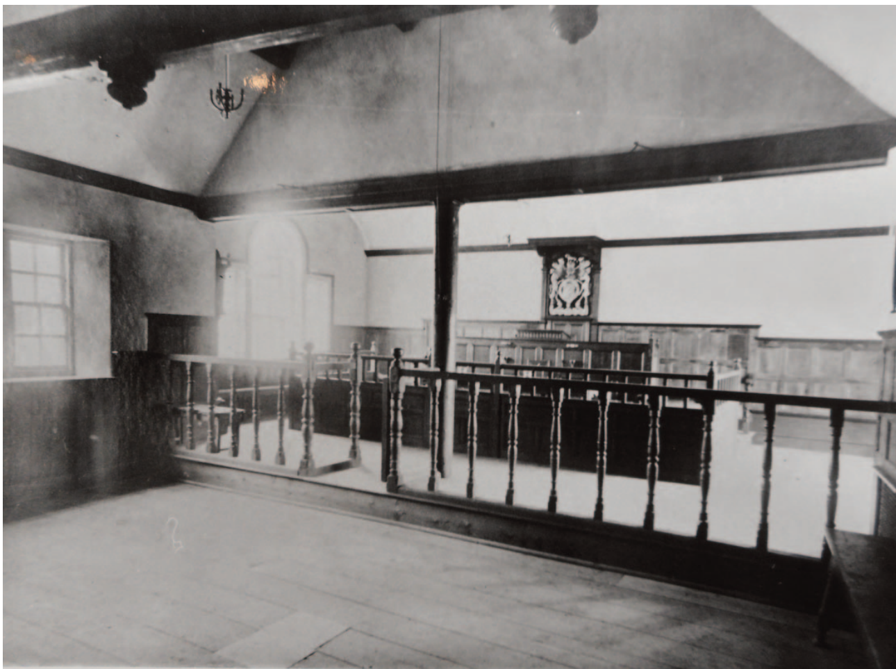
Fig. 34. The first floor of the guildhall after the works were completed. The plans show that the post supporting the ceiling beam was retained in-situ as was the step up to the court within this east bay.
