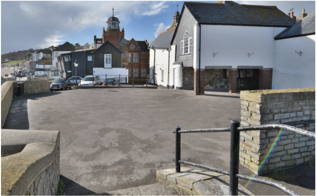
Fig. 19. The south elevation of The Guildhall with its angled eave and plain rendered facade where the adjacent cottages set on the lower ground beyond the railing were demolished.
