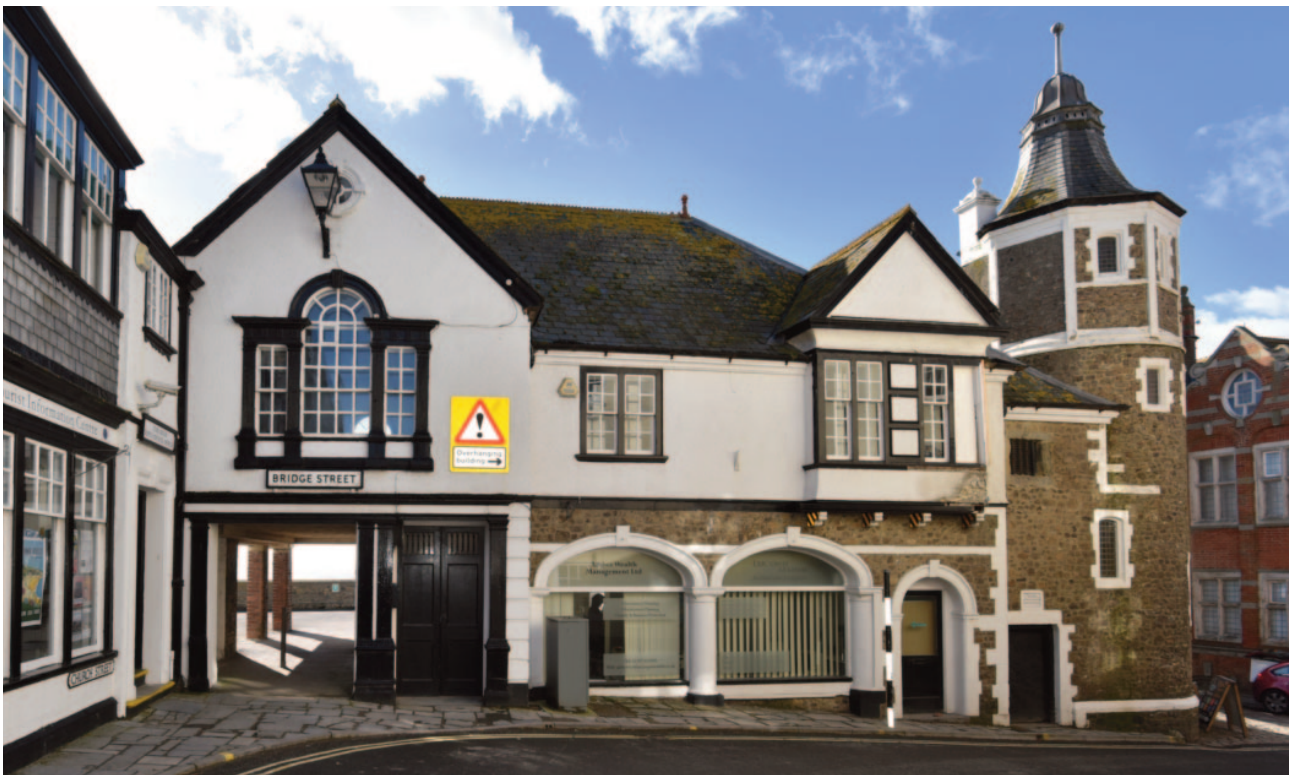
Fig 7. The front (north elevation of The Guildhall with its wide projecting gable to the left and the oriel window to the right. The two open ground floor bays to the left have been further opened up by removal of the east wall in the mid 20th century. Set back slightly on the right is the former jail and remodelled stair tower incorporating the main entrance porch. The left hand projecting bay may have survived the 1890 road widening.
