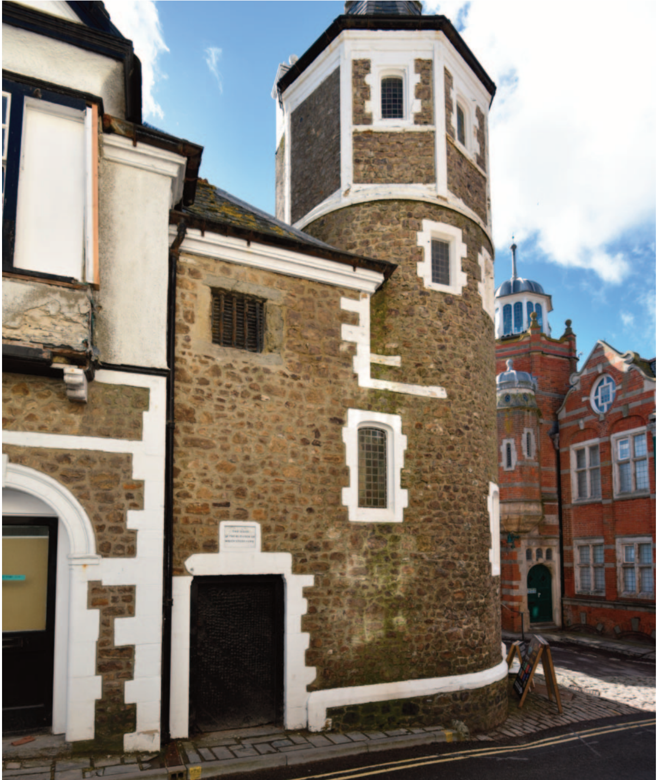
Fig. 9. The reformed north elevation of the former jail and guildhall, which was rebuilt behind its historic line to allow the road to be widened c.1890. It is unclear how much of the stair tower is historic.
