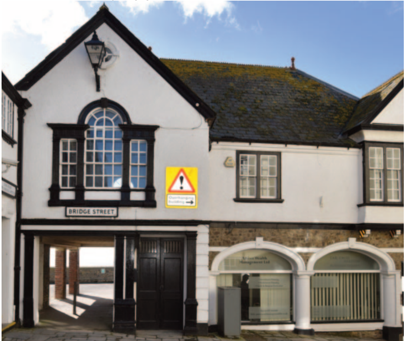
Fig. 11. The north elevation showing the possibly original left hand projecting bay with the refronted and set back central range with the former gaol and stair tower to the right.
