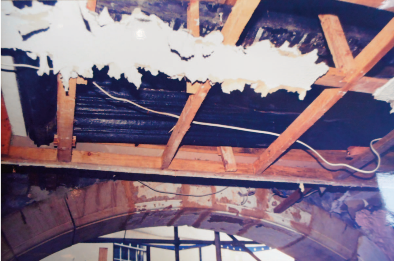
Fig. 21. The 16th century moulded ceiling beam surviving above the plaster ceiling in the ground floor of the guildhall. Exposed following vehicle damage in 1991 it shows charring from fire damage in the 19th century.
