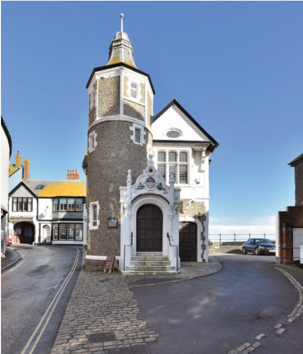
Fig.8. The west elevation with the ornate entrance porch containing the steps up to the first floor Guildhall and on the right the arched door to the ground floor rooms within the former market hall. Until the mid-20th century a row of cottages infilled the space between the Guildhall and the museum building on the right.
