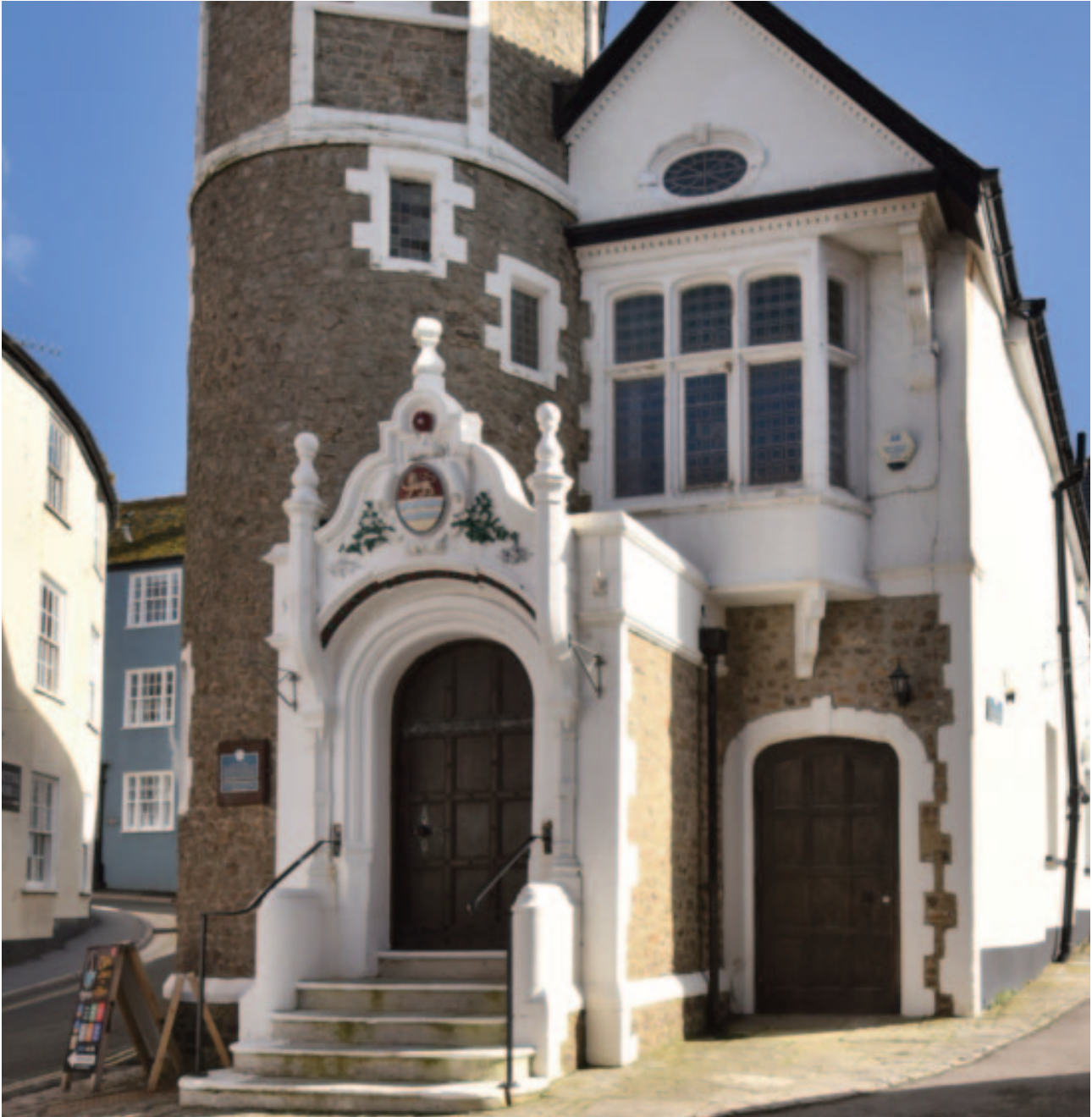
Fig. 16. The simply detailed raised front porch to the west elevation with the adjacent ground floor door to the right into what is now a separate office.
