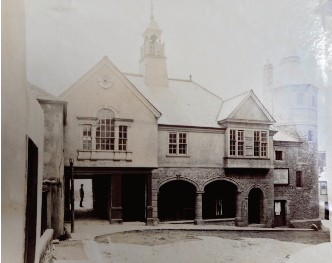
Fig. 29. The guildhall following the Vialls work in the late 19th century. The open walkway to Gun Cliff and the adjacent entrance to the open market area below the guildhall can be seen on the left, with the open arches to the market on the right. The adjacent door is on the site of the former entrance door to the guildhall stairs but following the rebuilding it opens into the open market area .
