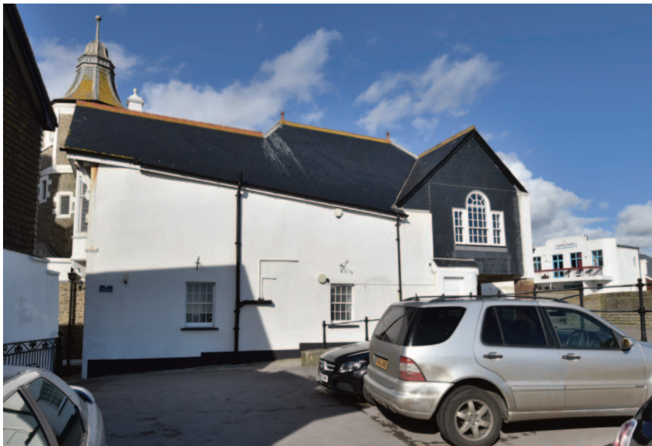
Fig. 18. The more simply detailed south elevation with its angled eave and plain rendered facade was originally attached to historic cottages which were set on the lower ground in front of the railings.
