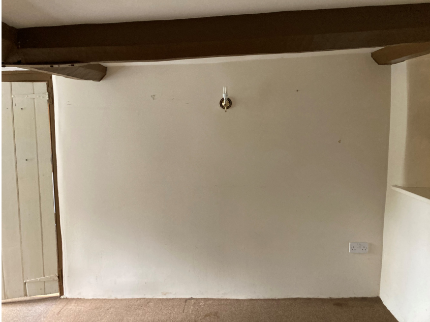
Wall between kitchen and dining room to be removed
