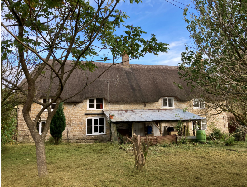
Southern elevation – lean-to extension to be replaced
