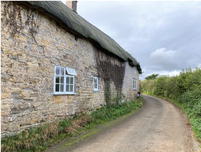
Northern elevation – historic window openings to be reinstated
