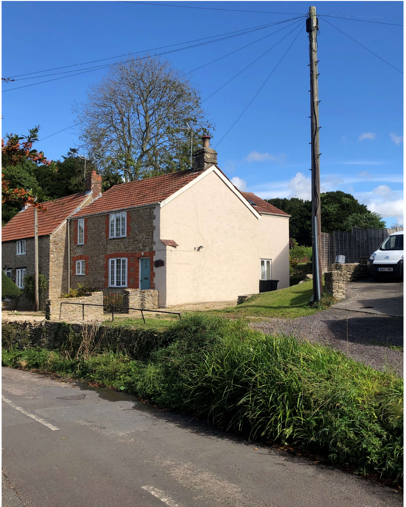
Figure 3: This Property (shown on the map as 1) has been extended in a very similar fashion as proposed here, the eaves are higher than the existing building however the ridge line is lower and being set back it still achieves subservience. This house is in a prominent location on Rectory Lane, clearly visible as you enter the village from the coast road.
