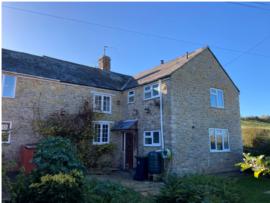
Rear elevation – location of the two storey extension.
