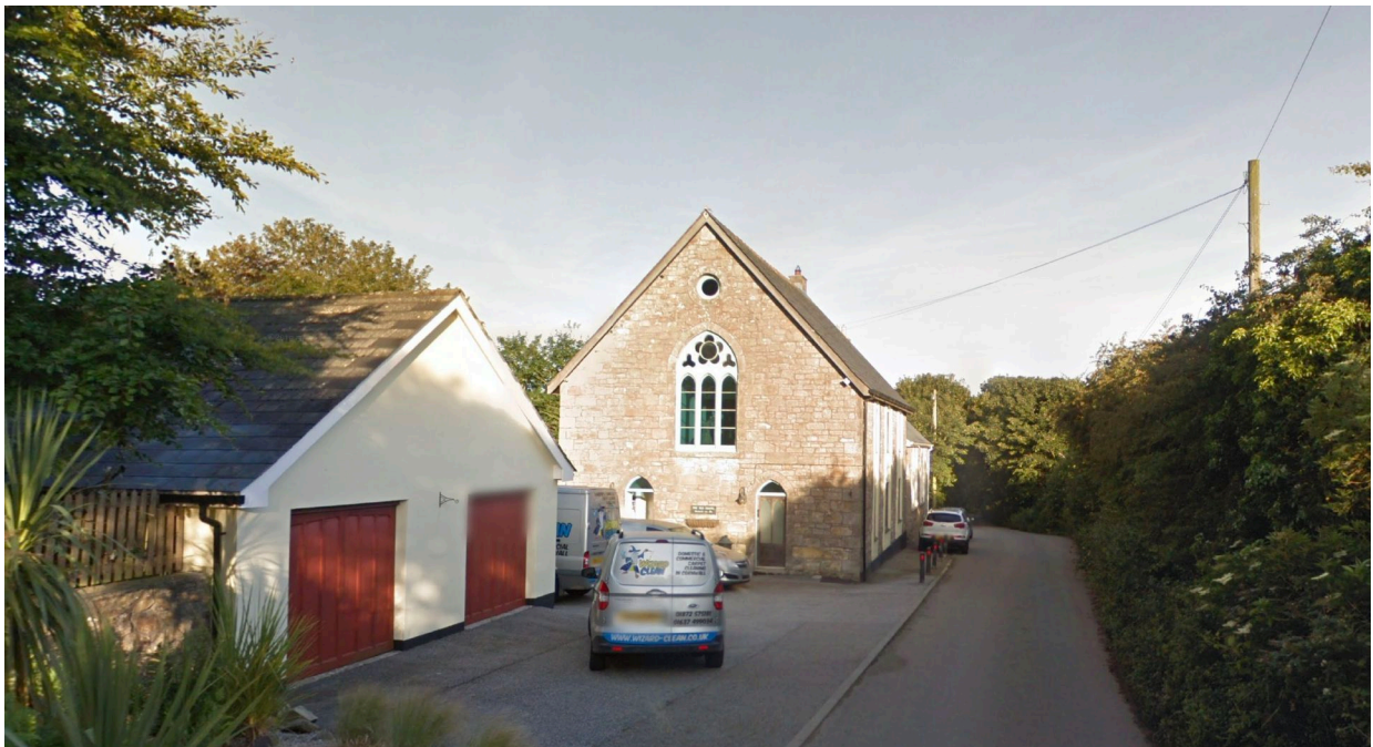
Old Chapel and Old Sunday School (as designated on Ordnance Survey ) is the property to east of side - with lower level garage.
