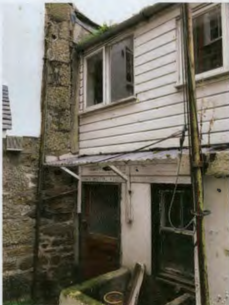
Back of property showing the weatherboarding and door which it is proposed to replace and the remains of the coal store.
