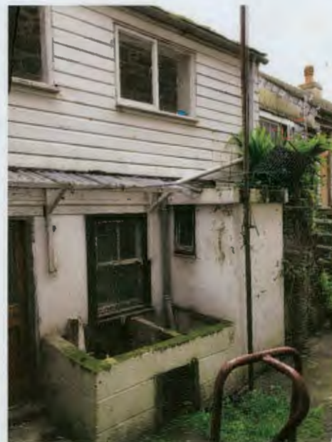
Back of property showing the weatherboarding and door which it is proposed to replace and the remains of the coal store.
