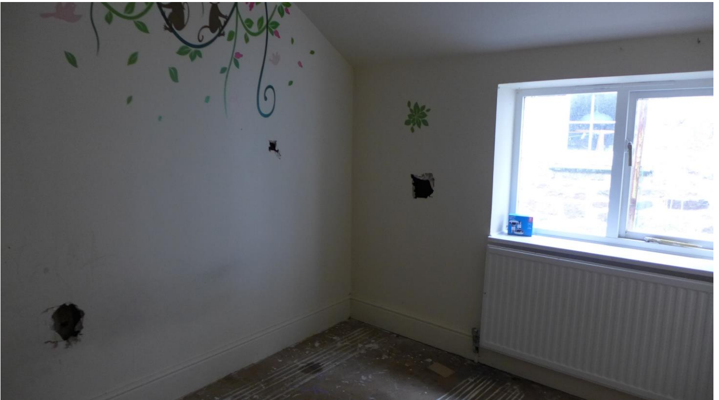
Figure 3. Interior of a room on the upper floor.
