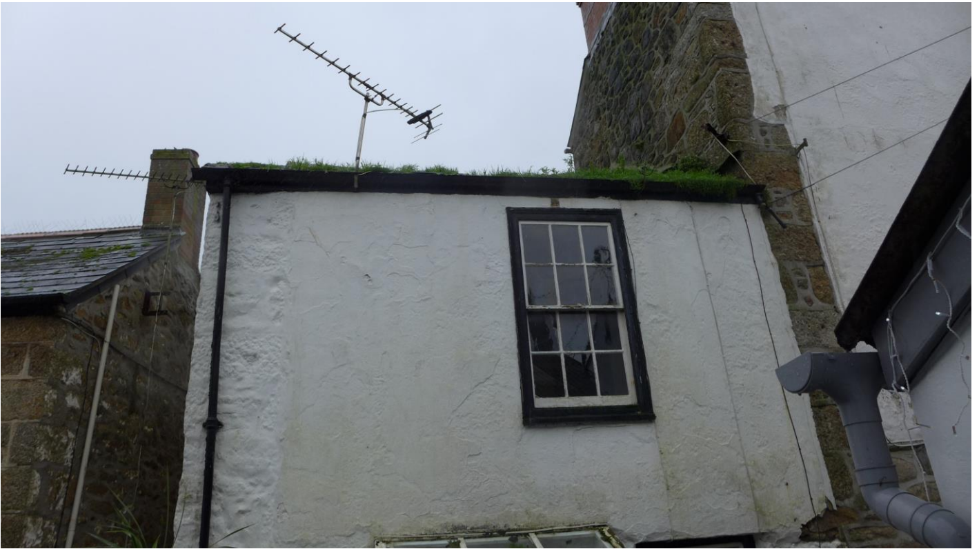
Figure 2. Upper floor, eastern aspect.
