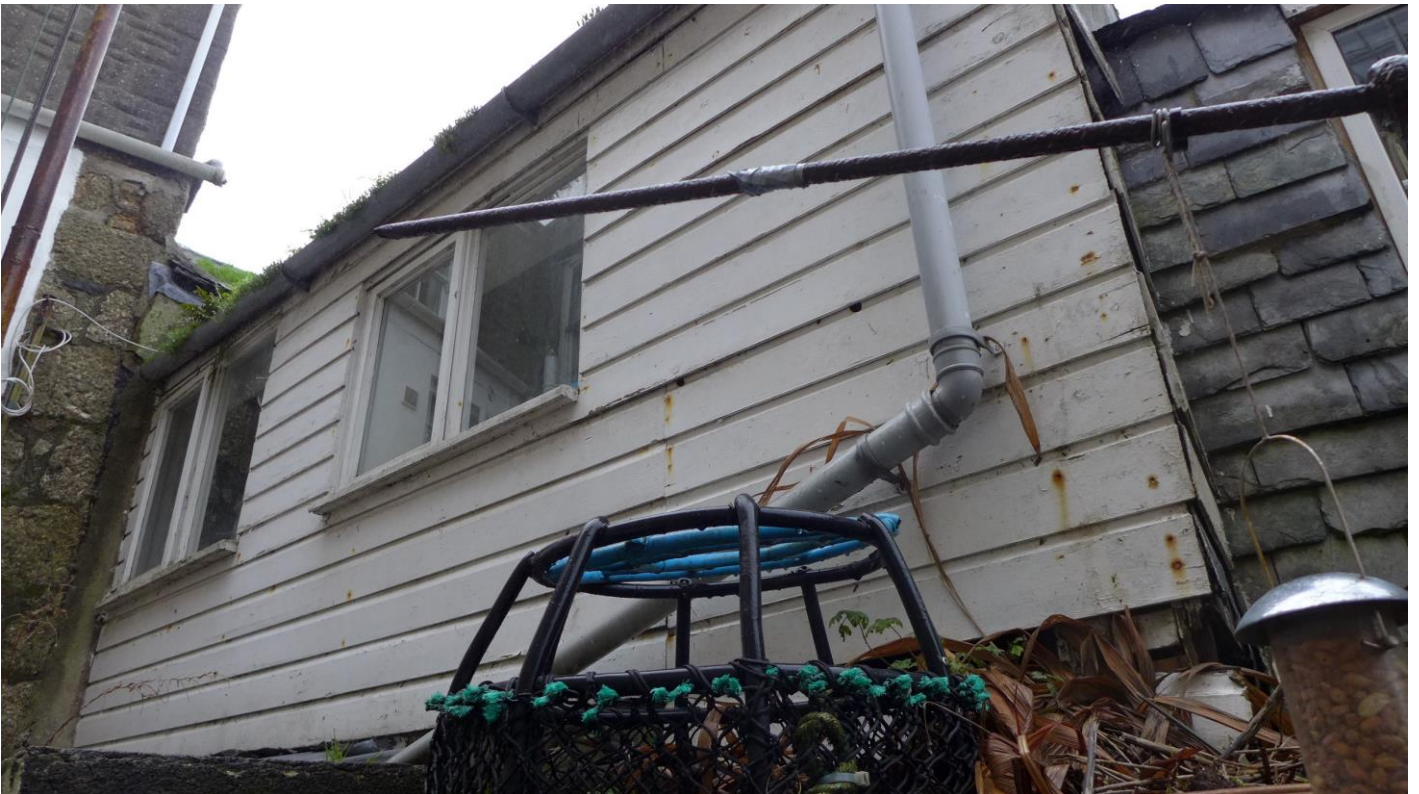
Figure 5. Weatherboarding on the western aspect, upper floor.
