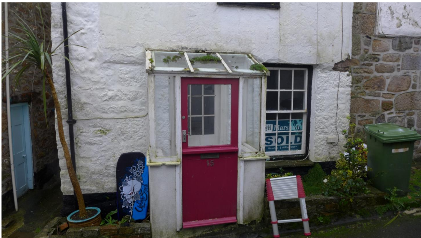
Figure 1. Main entrance to the property, eastern aspect.
