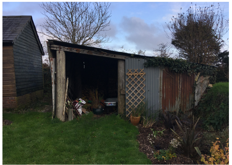
Fig.4 photograph of outbuilding next to workshop
