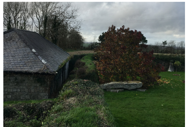
Fig.5 photograph looking westward at garage with garden hedge in foreground
