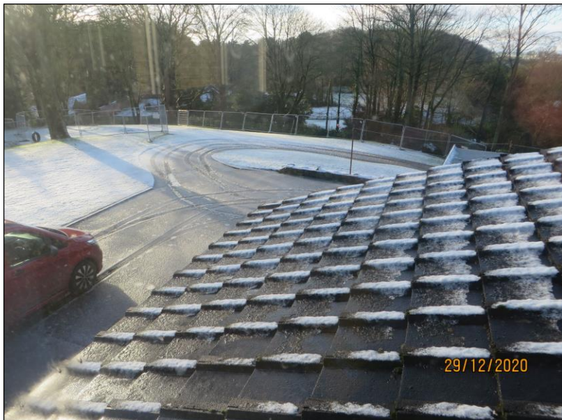
Figure 14. Single-storey roof viewed from upper floor window.
