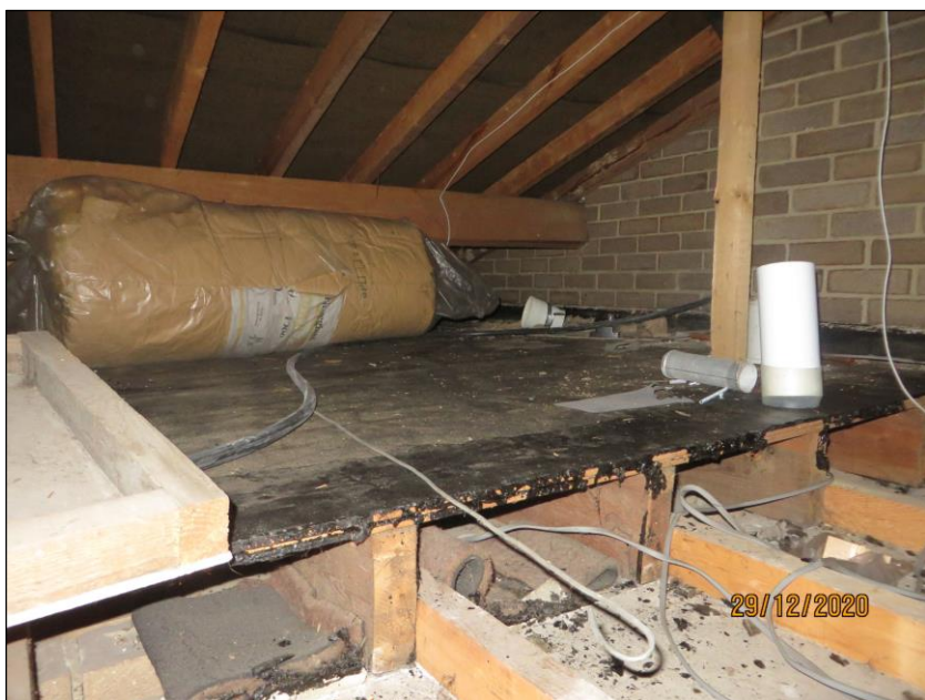
Figure 16. Single-storey loft void.
