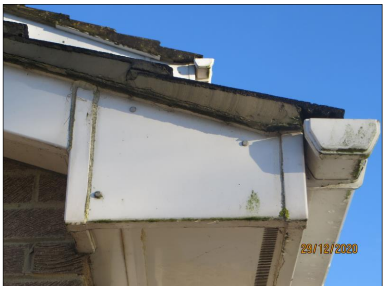
Figure 13. Soffit boxes in a good state of repair and flush to the wall.
