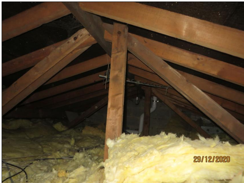
Figure 17. Main house loft void.
