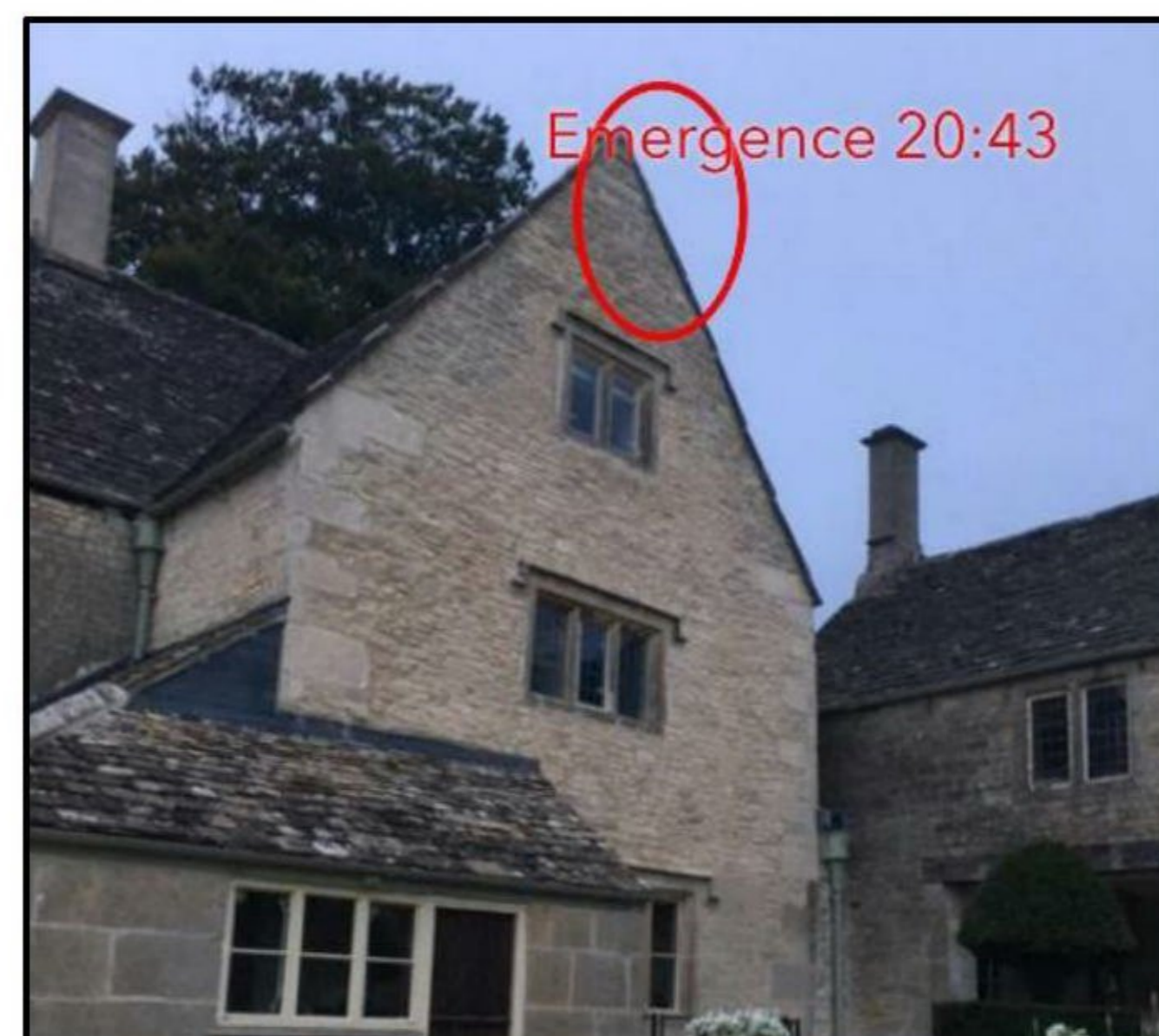
Photo 17: Emergence location of building west of B1 not impacted
