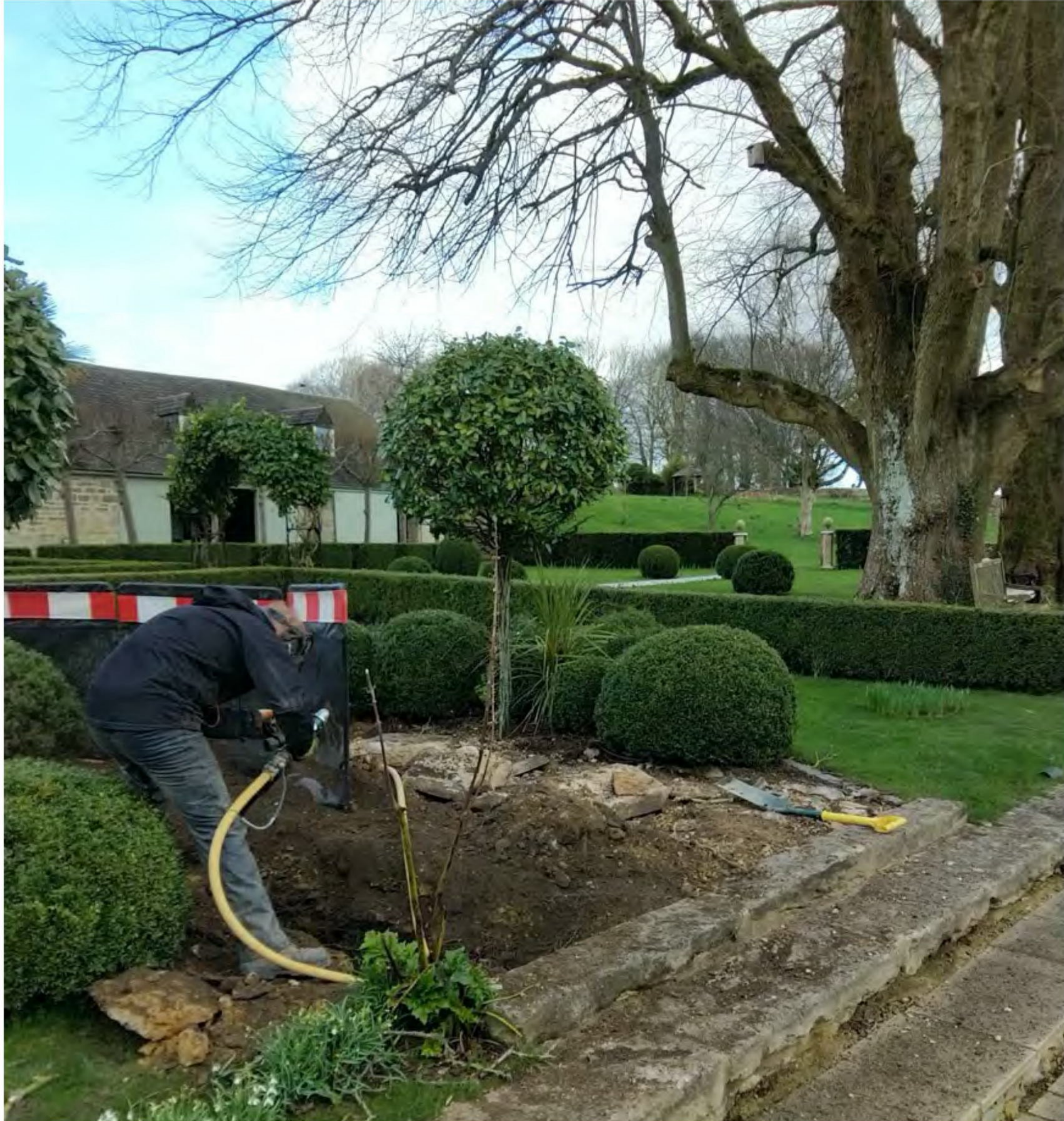
Image 6: Showing the location where the second trial trench was excavated as part of further investigation. The image shows the proximity of the adjacent lime to the area where the new extension is proposed (approx. 10m between stem and closest edge of the trial trench).
