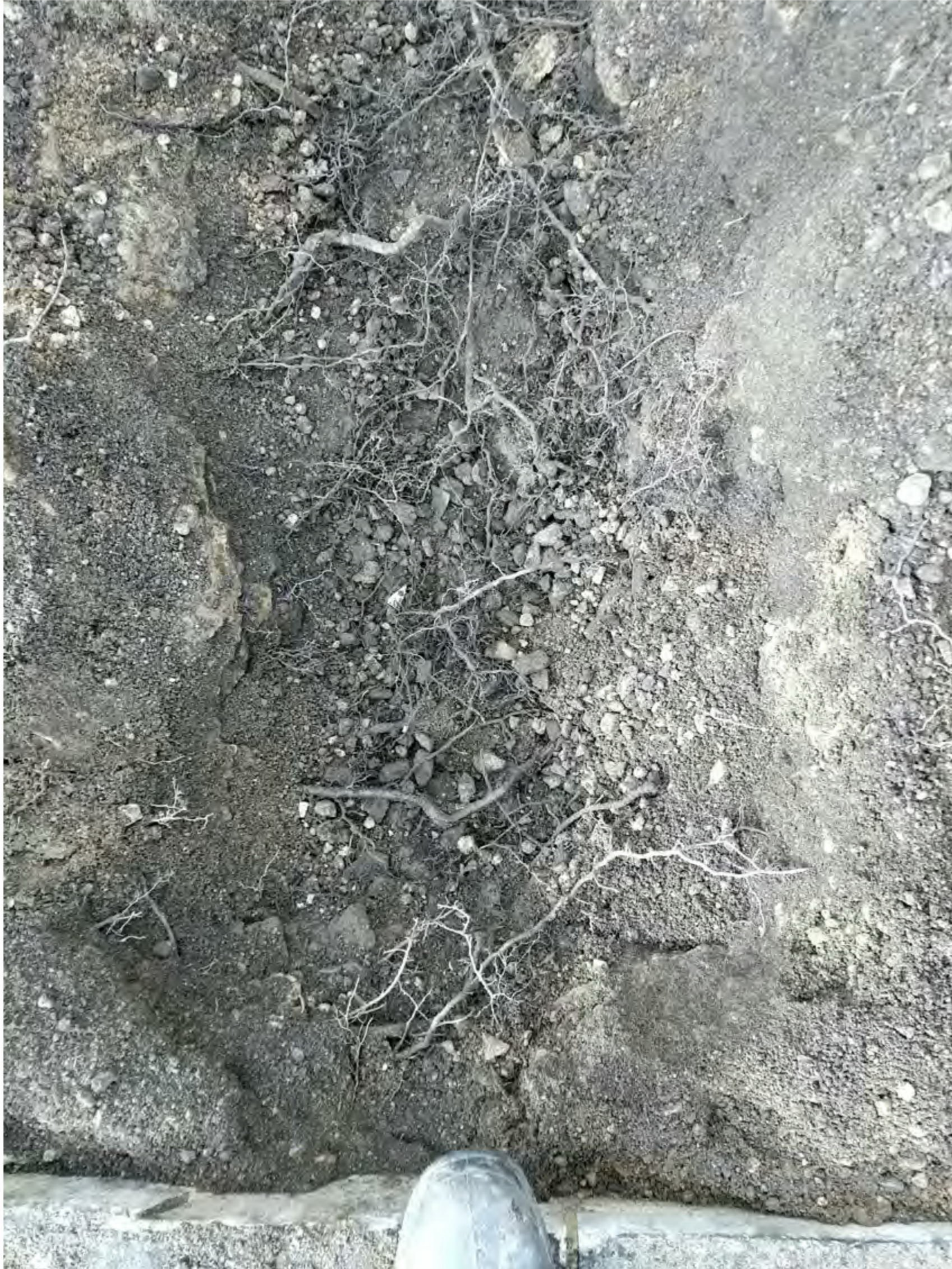
Image 7: Showing the southern section of the trench with the retaining wall visible at the bottom of the image. 'Section 1' of the trench open with the gravel and top 400mm of soil removed showing a sparse concentration of fibrous root and some small diameter (10mm) feeder roots present.
