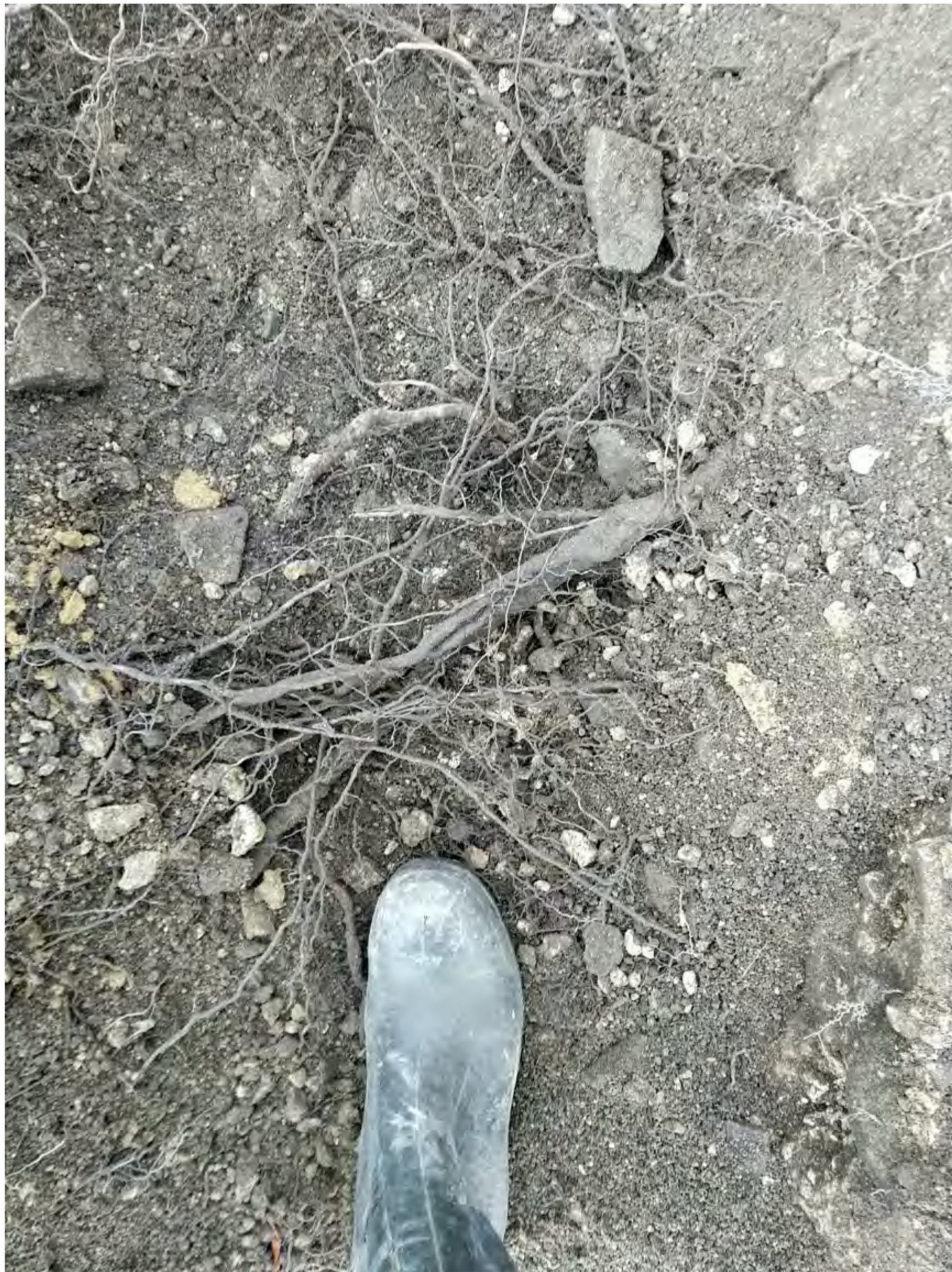
Image 8: Showing the northern portion of 'Section 1' of the trench open with much of the stony and made up ground removed with a single slightly more significant feeder root of 30mm and the associated fibrous root growth present.
