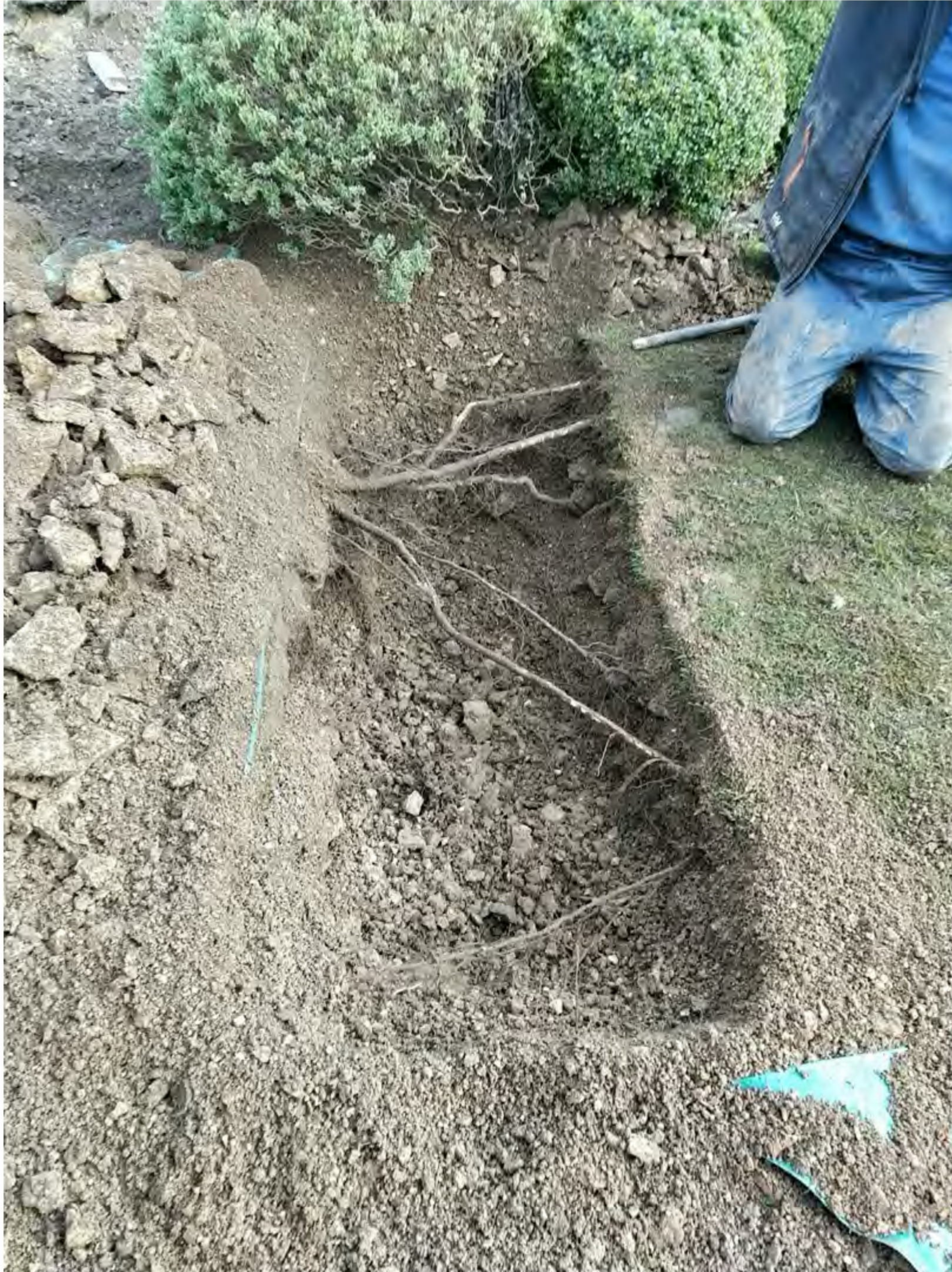
Image 9: Showing 'Section 2 of the trench open with much of the stony and made up ground removed and a root of 25mm and some fibrous root growth present.
