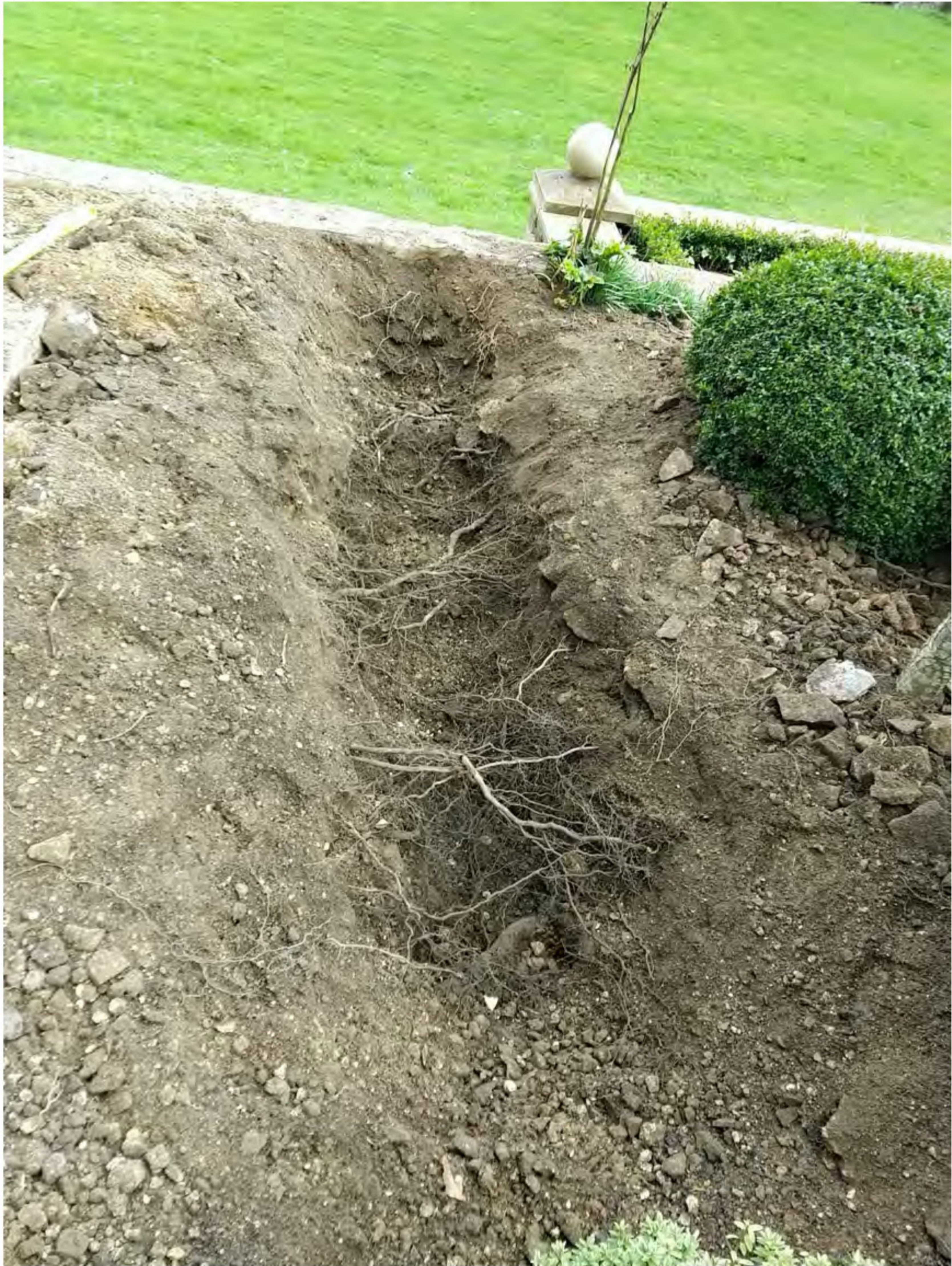
Image 9: Showing the full extent of the first 3m trench fully excavated to approx. 500mm. A lower density of fibrous and feeder root than the initial trench with only one more significant root visible at the northern end of the trench which was approx 50mm diameter.
