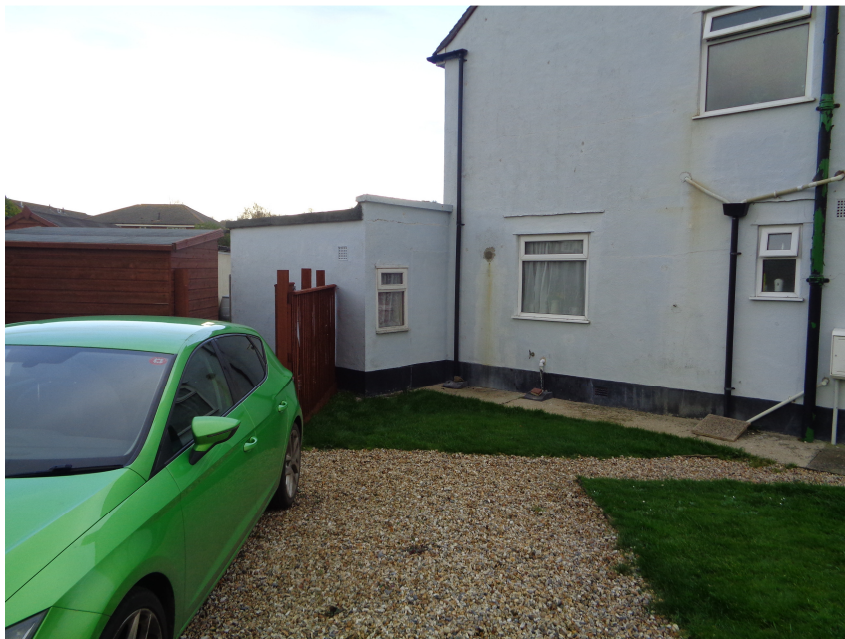
Close up of NW Elevation
