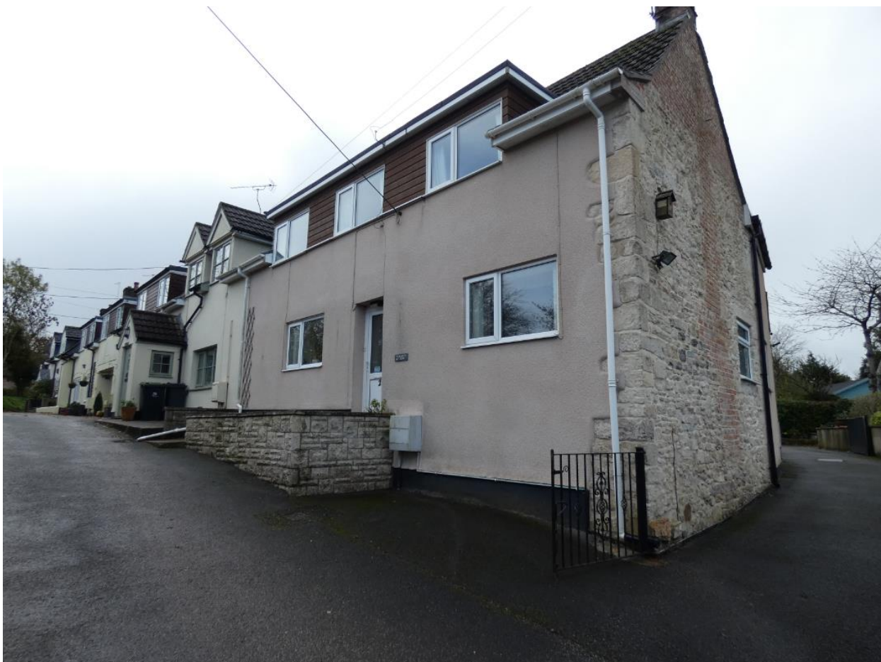
Photo 1 – North East Elevation (Front) Existing porch to no. 3 Hardy's Row visible in background.
