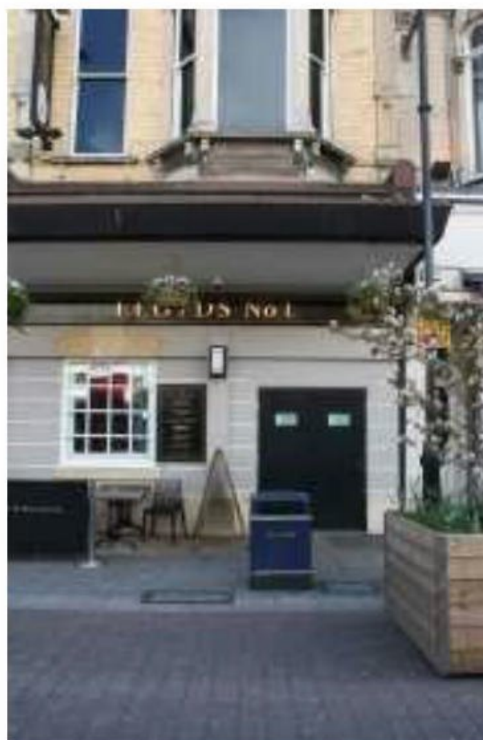
The current service / escape access will become the dedicated Hotel Guest entrance
