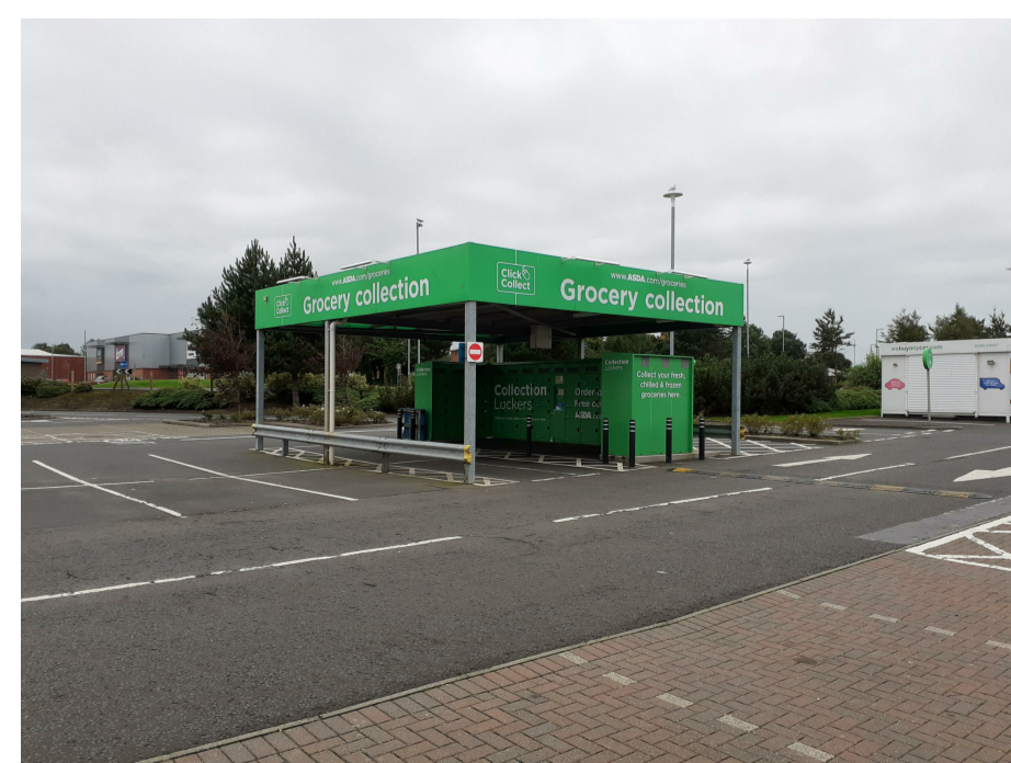
Existing C&C Canopy - Photograph P1
