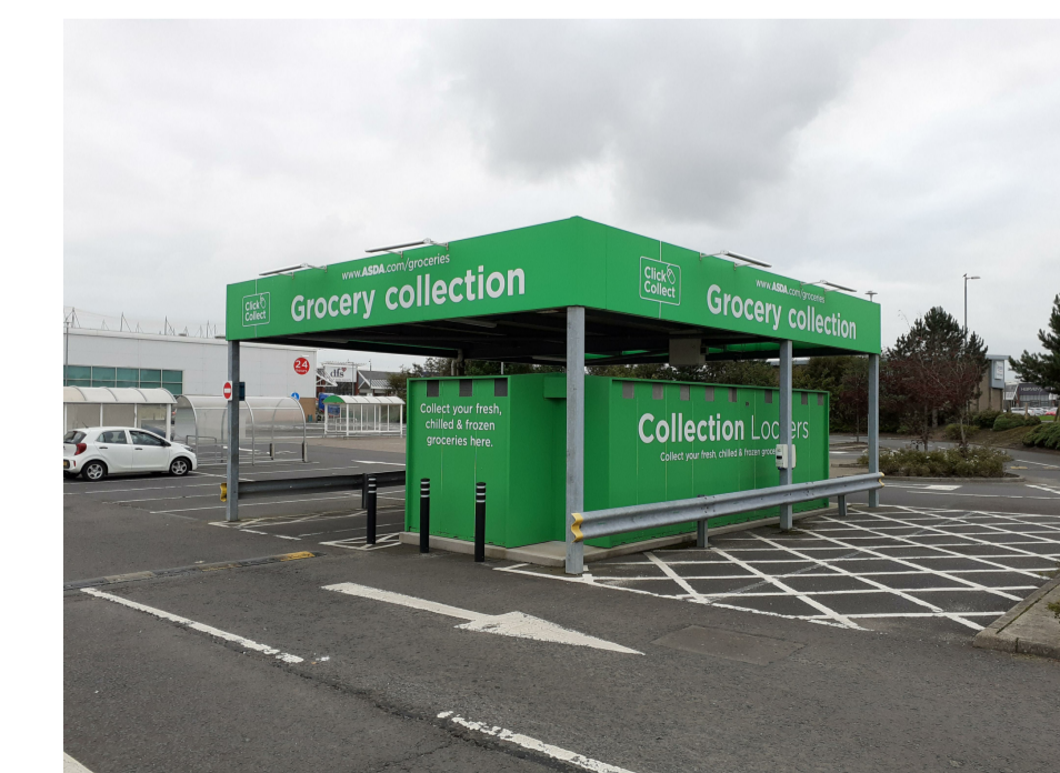
Existing C&C Canopy - Photograph P2
