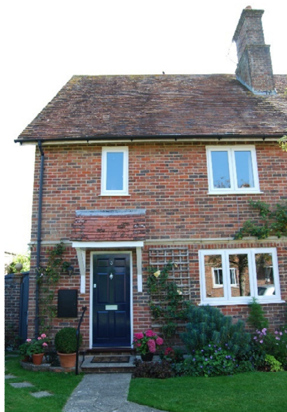
View of West Elevation.
