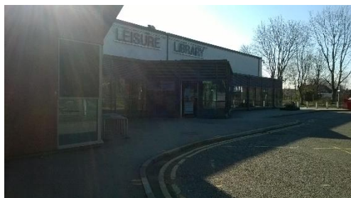
Figure 2: North elevation of building
