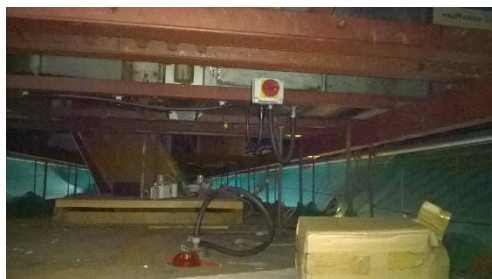
Figure 8: Void above swimming pool
