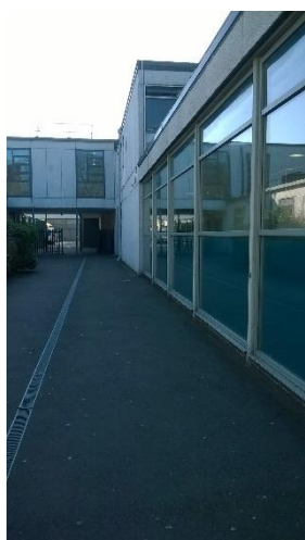
Figure 4: Bridge on east elevation
