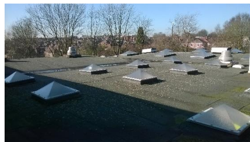
Figure 9: Roof of building
