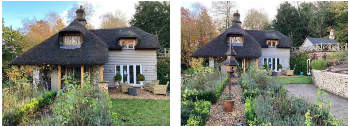
Figure 3 East Elevation to Swarraton Lodge
