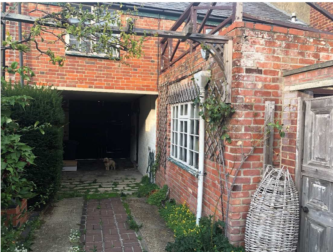
Undercroft viewed from rear driveway
