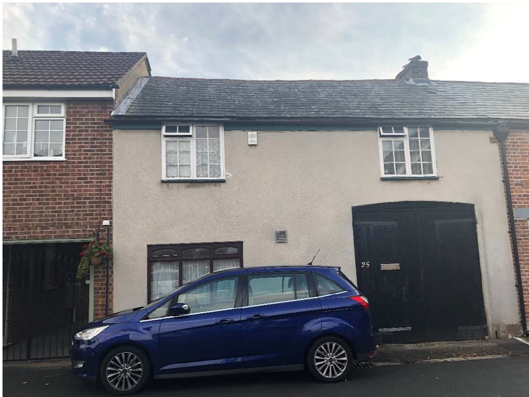
front elevation showing old coach entrance doors
