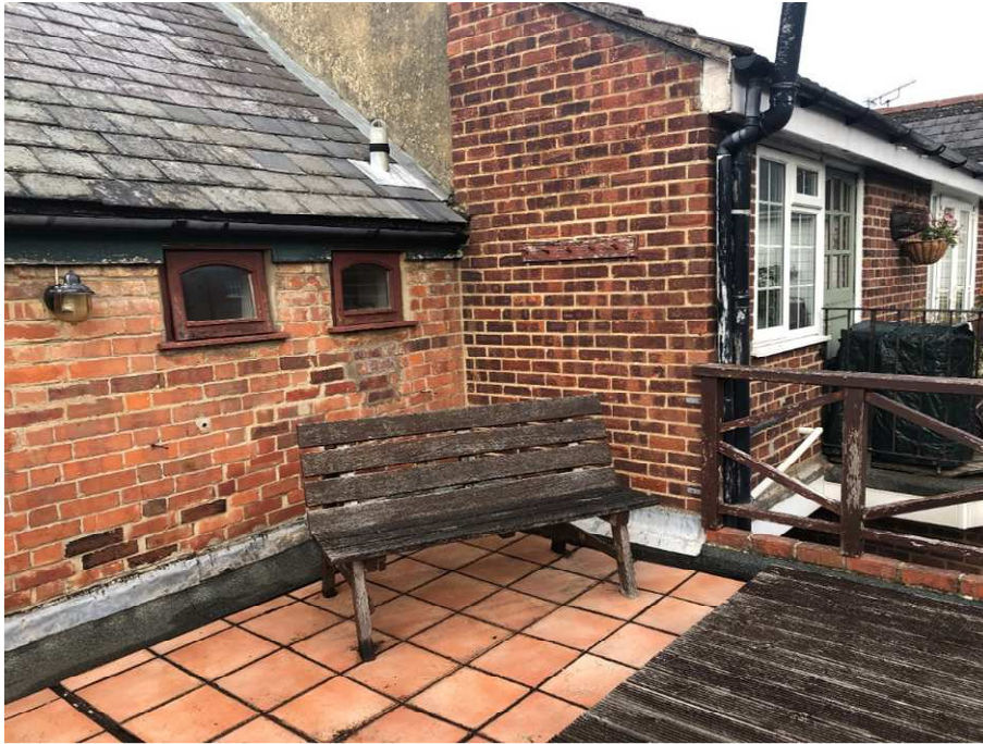
existing first floor patio terrace
