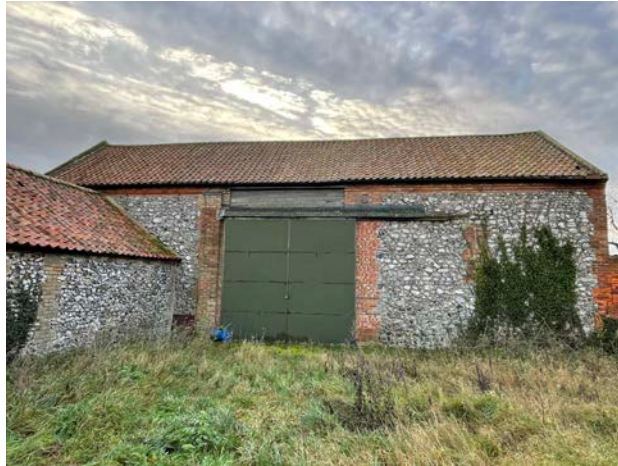
Photo 4 - Rear / north elevation
