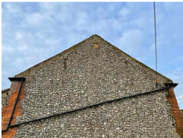
Photo 2 - Right / east gable
