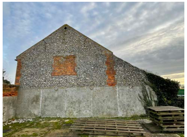
Photo 3 - Left / west gable
