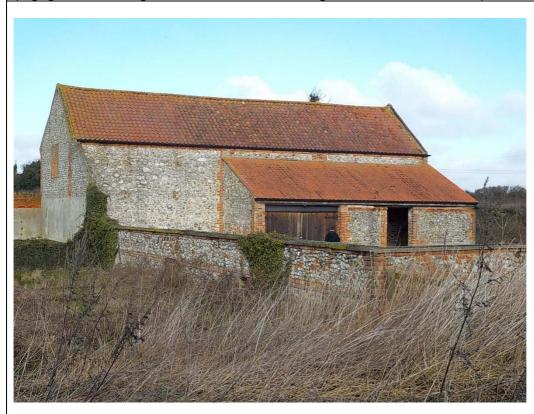
The property has brickwork and stone visible externally with timber doors with Clay Pantile roof tiles over with UPVC gutters and downpipes. The outside ground is hardstanding / concrete access with grassed areas to the sides and rear. The building is used for storage of farm equipment with no visible signs of contamination.
