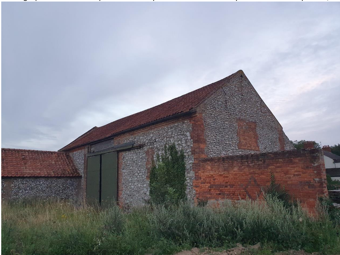
Photograph 2: Western and northern aspects of barn
