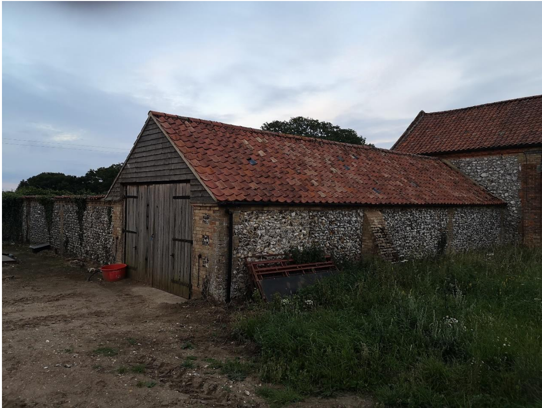
Photograph 3: Northern and western aspects of single storey extension
