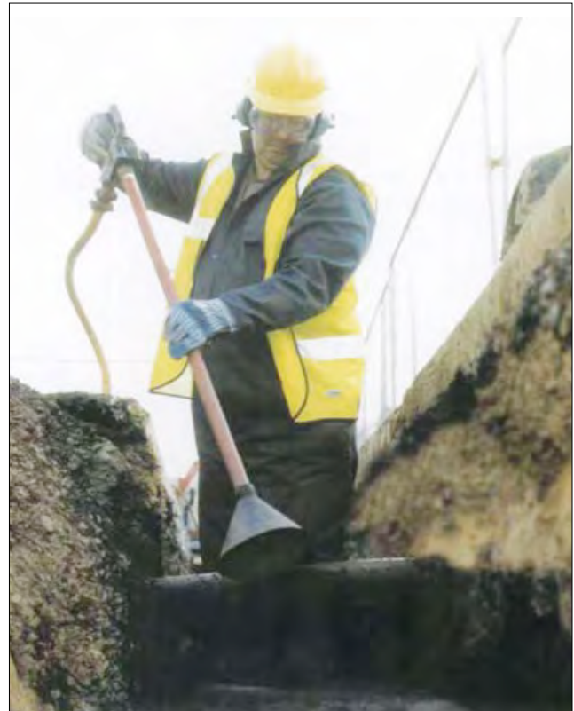
Figure 7 Using an air digging tool
