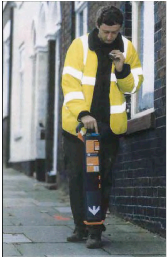
Figure 5 Using a cable locator
