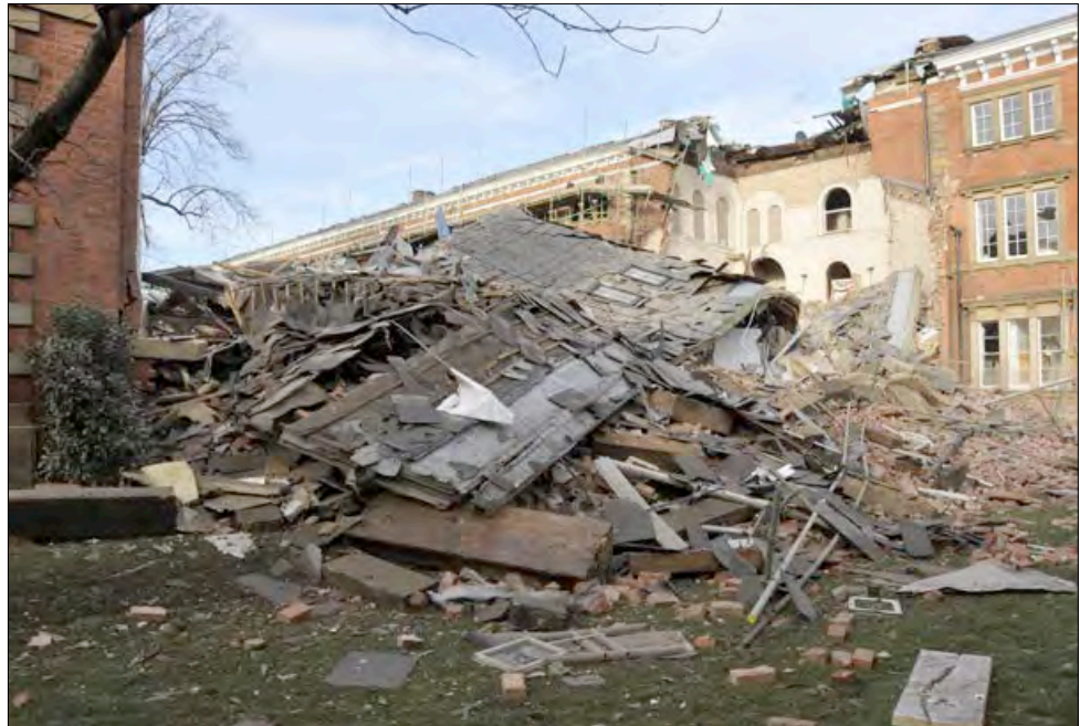
Figure 1 Aftermath of a gas explosion, following damage to an underground gas service pipe
