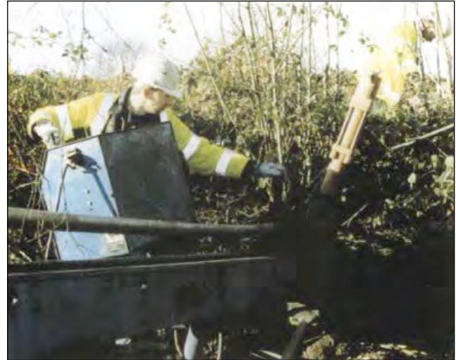
Figure 8 Horizontal drilling being used for laying a cable under a road
