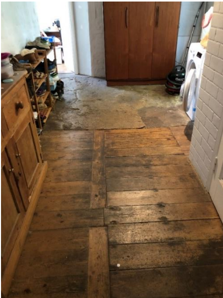
Fig. 1 photo of the current utility room area.
