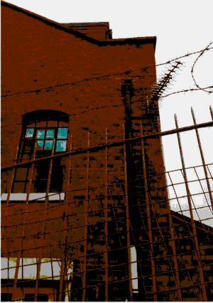
Unit 7, Block B, 2 Fawe Street (PA/11/01152/A1)
