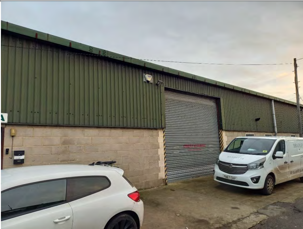
Photo 1: View looking southeast towards the western façade of the building on-site.
