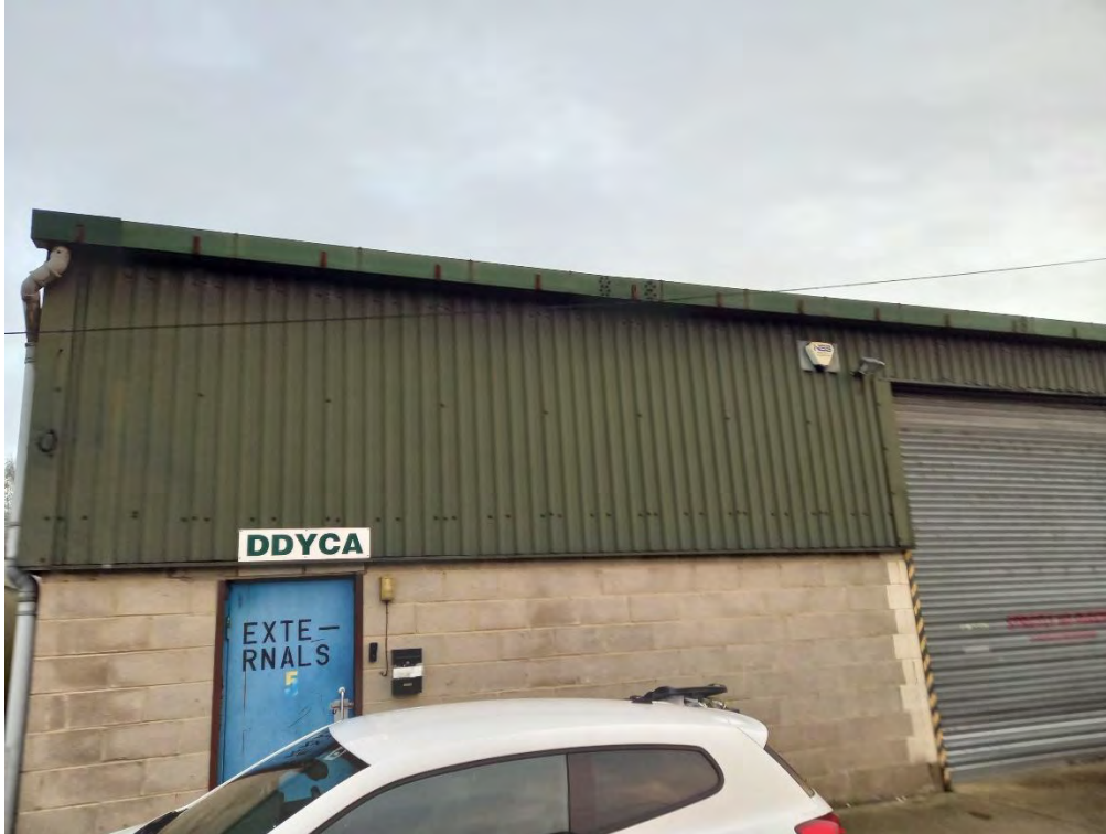
Photo 2: View of the northwestern corner of the building, looking east.
