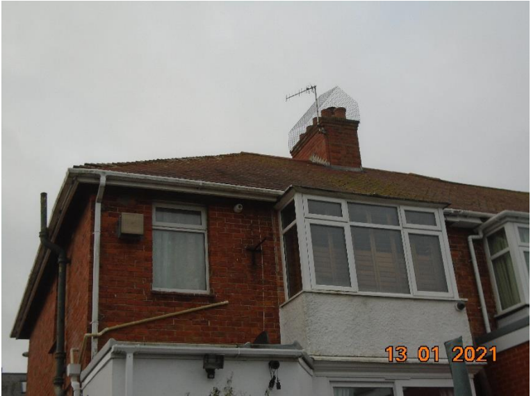
Photo 2: Northeast elevation of house
