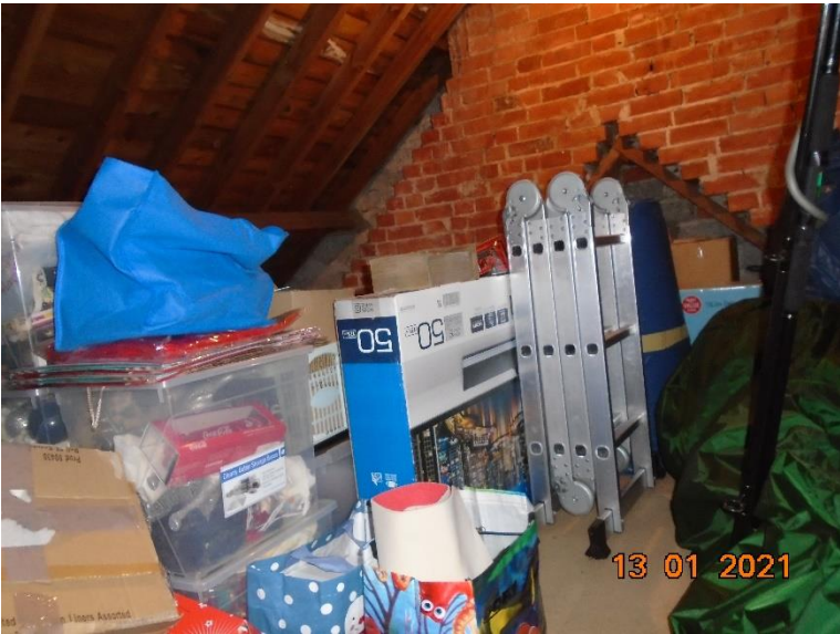
Photo 3: Internal loft void of house
