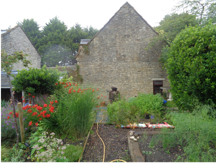
Existing southern elevation identifying former opening
