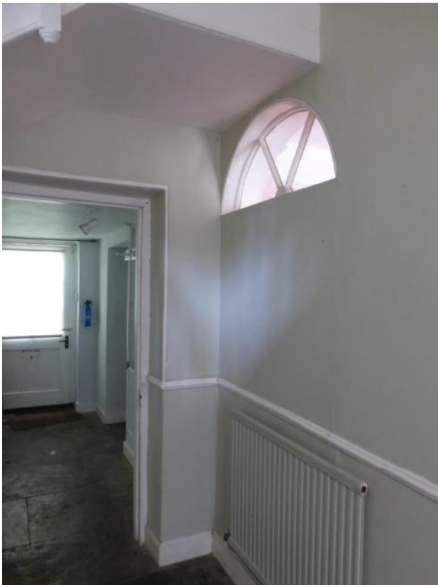
Fig.5 Fanlight over the blocked original doorway into the rear service wing.
