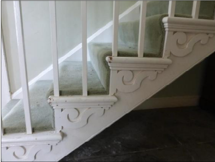
Fig.7 Scrolled stair tread ends.
