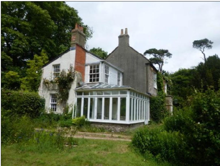
Fig.2 The South-West elevation showing the original gable (now rendered) end of the house, the extension of the rear range and the 20 th century conservatory and timber first floor extension.
