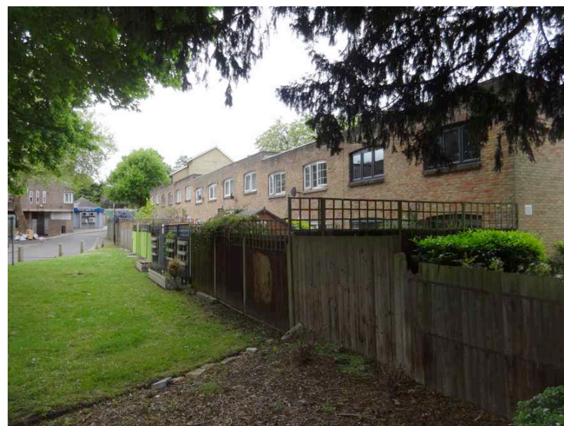
Rear elevation in the context of its neighbours
