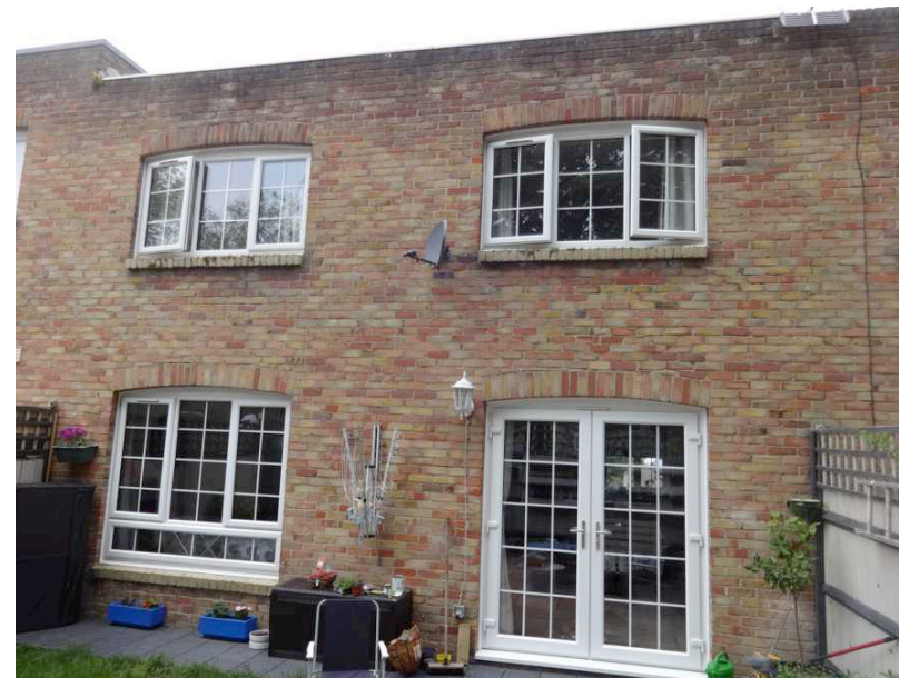
Rear elevation no.2 Limetree Close
