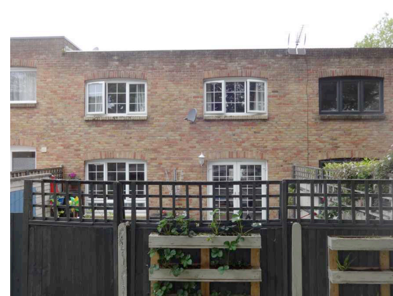
Rear extension and immediate neighbours
