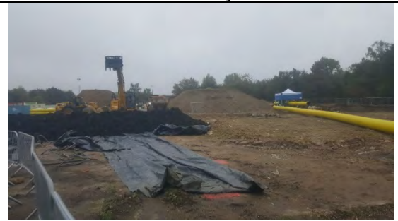
Visqueen ready to be placed over pile at end of day
