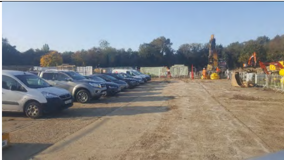
View of car park with new car park in background
