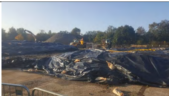
View of covered biopiles with crushed concrete stockpile in background
