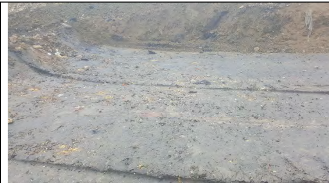
Rolled in material pre crush concrete 'firm clay'
