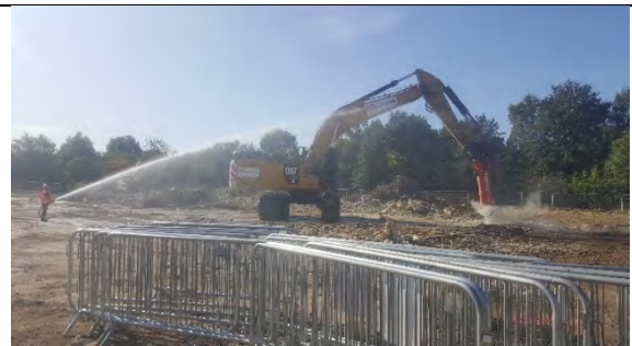
50t excavator, dust suppression breaking out concrete
