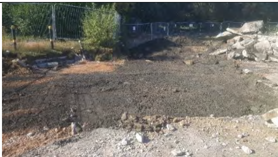
Blackend soils exposed at southern end of site whilst looking for rising main entry
