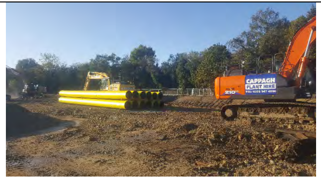
Stockpiled pipework awaiting installation
