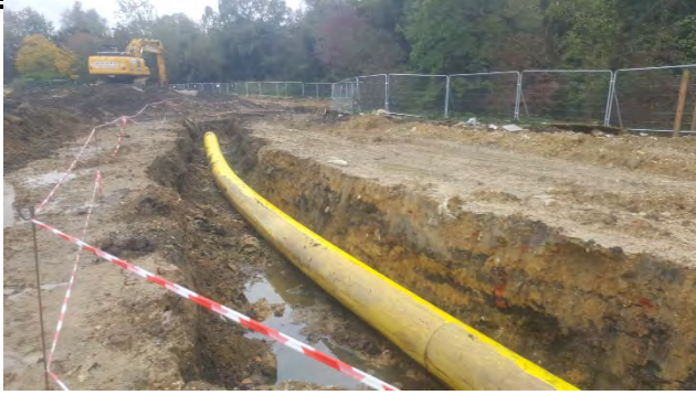
Gas main starting to be laid
