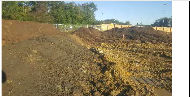
Mounded arisings from gas trench
