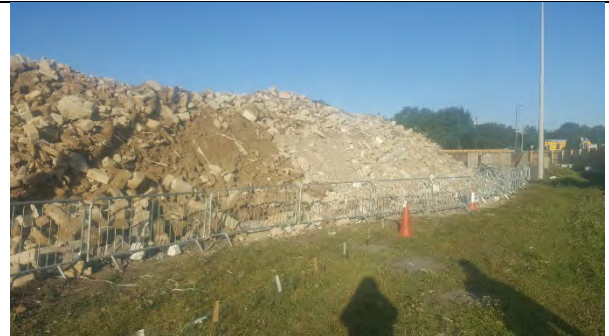
Sorted concrete ready for crush
