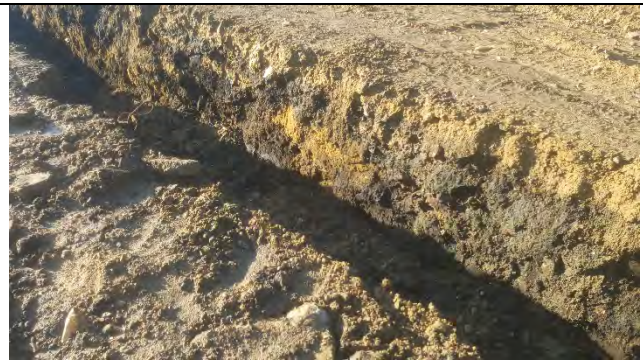
View of gas trench, c1.5m depth
