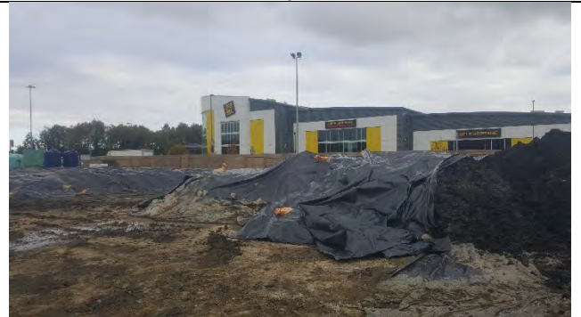
Biopiles covered in visqueen
