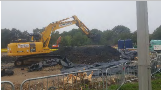
1 st biopile being turned by riddle bucket
