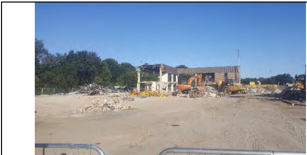
View from compound of remaining buildings
