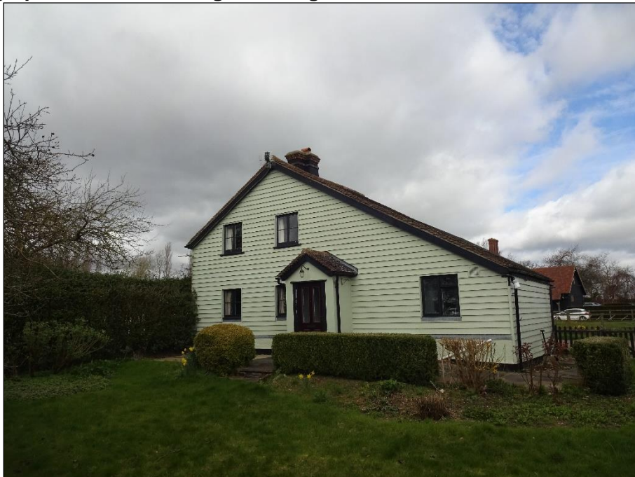
Photograph 2: Front of cottage, looking north. 11 th March 2020.
