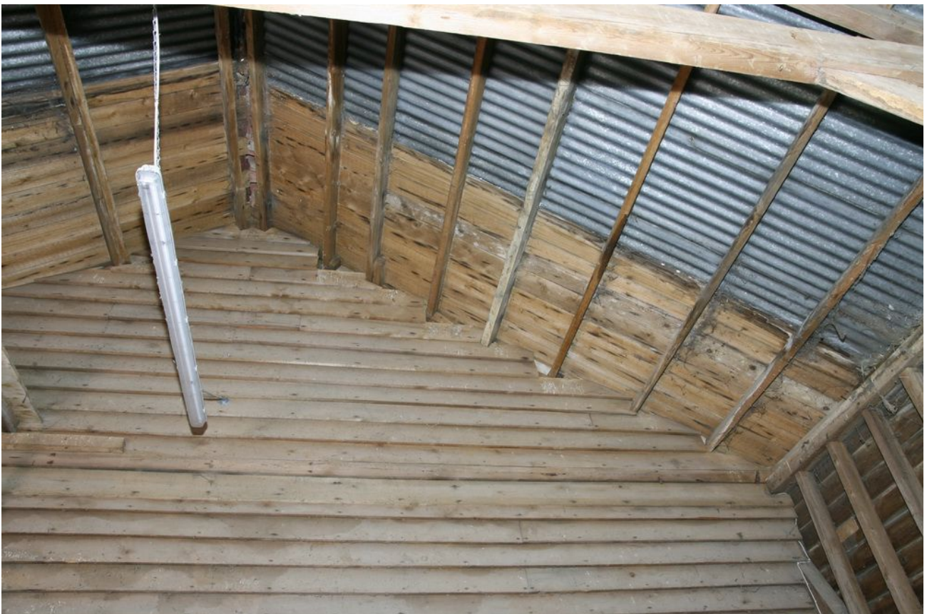
Plate 06 - Roof structure at junction between barn and cottage, looking S
