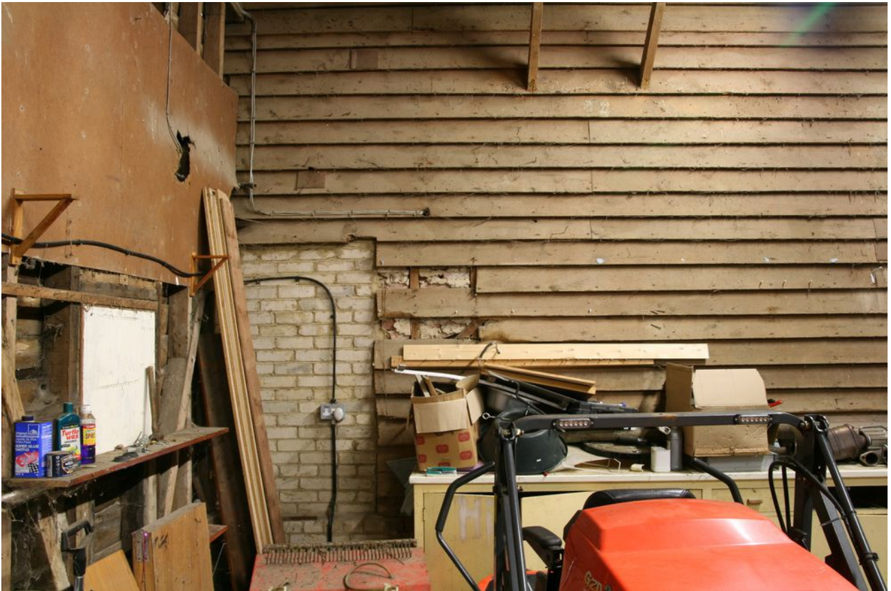
Plate 11 - Exposed framing and blocked door in S elevation, looking S
