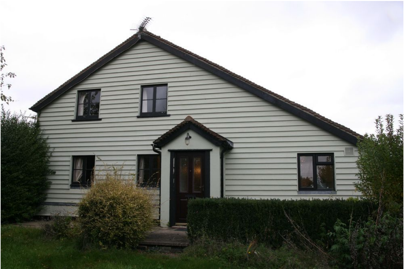
Plate 03 - Southern exterior elevation of cottage, looking N
