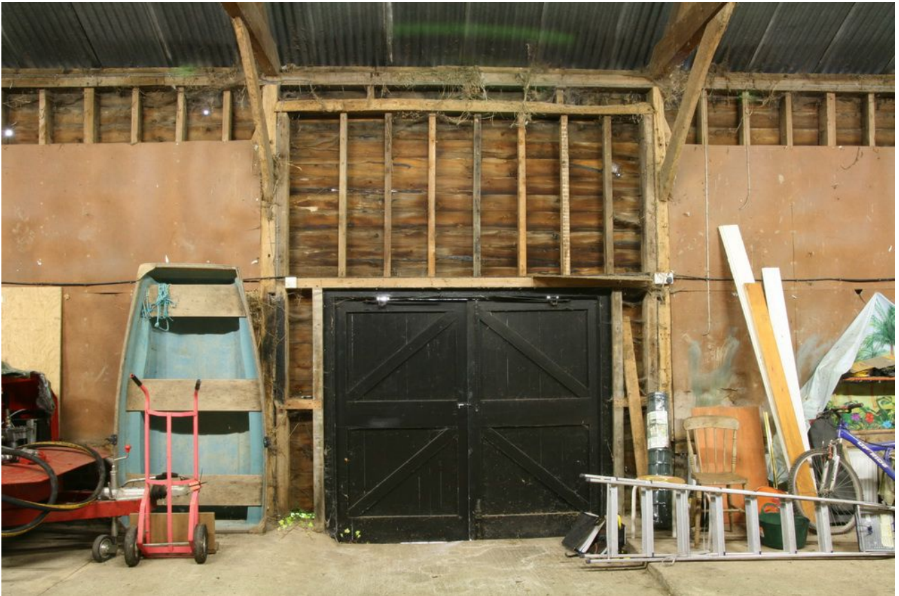
Plate 07 - Eastern barn door opening, looking E
