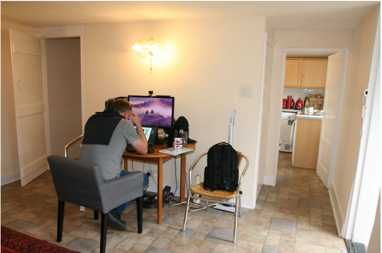
Plate 13 - Stair and kitchen access, E ground floor, looking ENE
