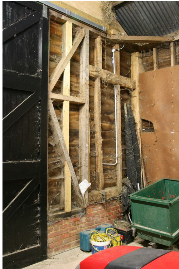
Plate 09 - Early framing in NE corner of barn, looking NE
