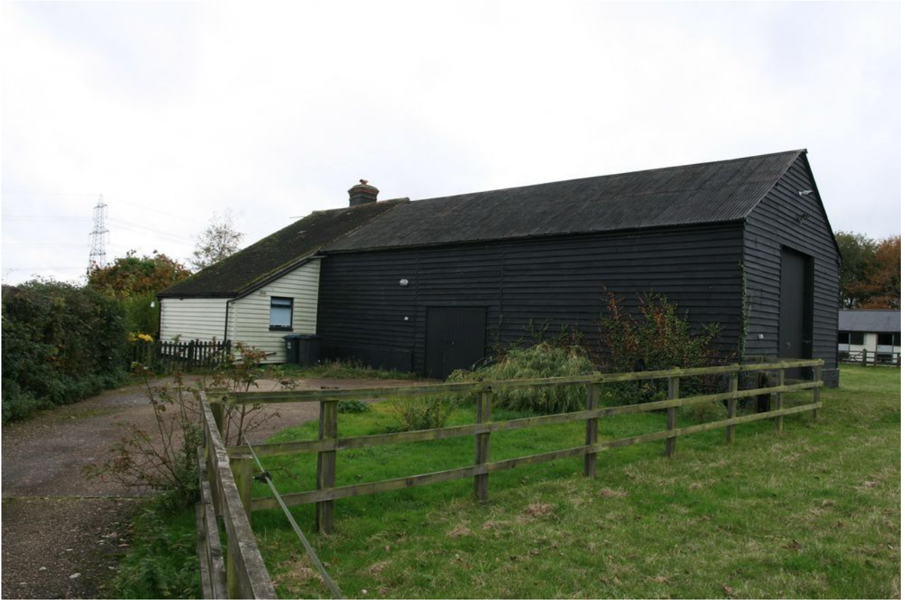
Plate 01 - View of cottage and barn, looking SW
