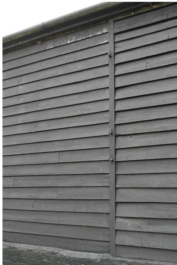
Plate 02 - Pintles in north jamb of blocked western doorway
