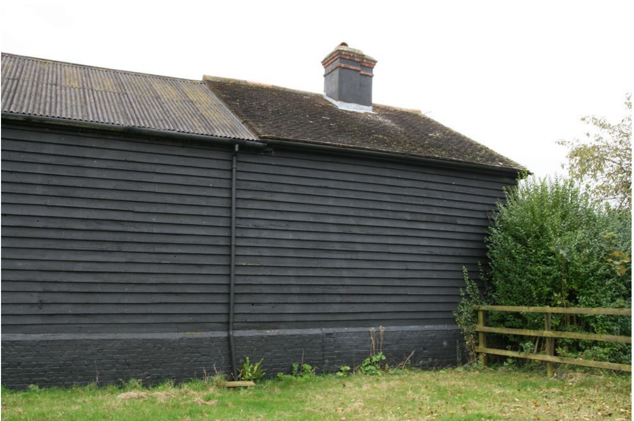
Plate 04 - Chimney and roof to cottage and barn, looking SE
