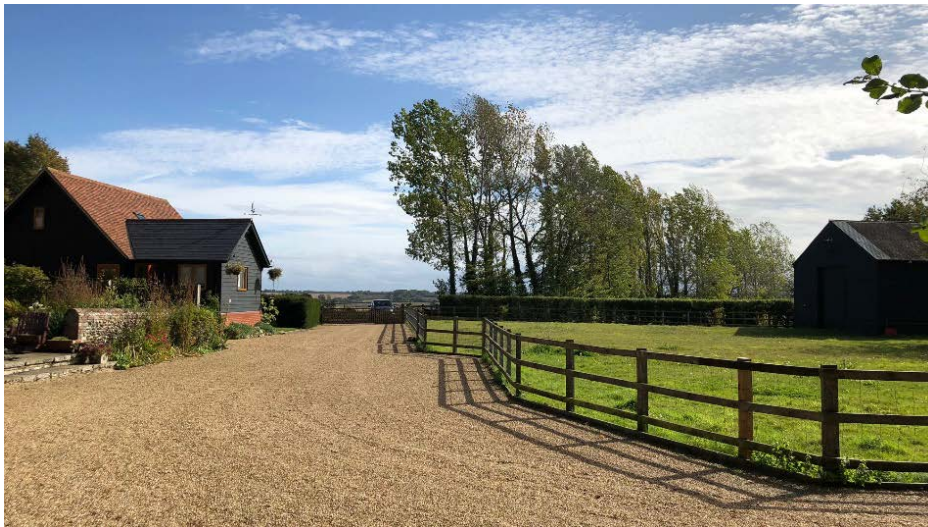
Figure IV – View across existing shingle driveway.
