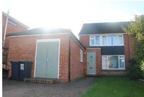
Single storey side building
