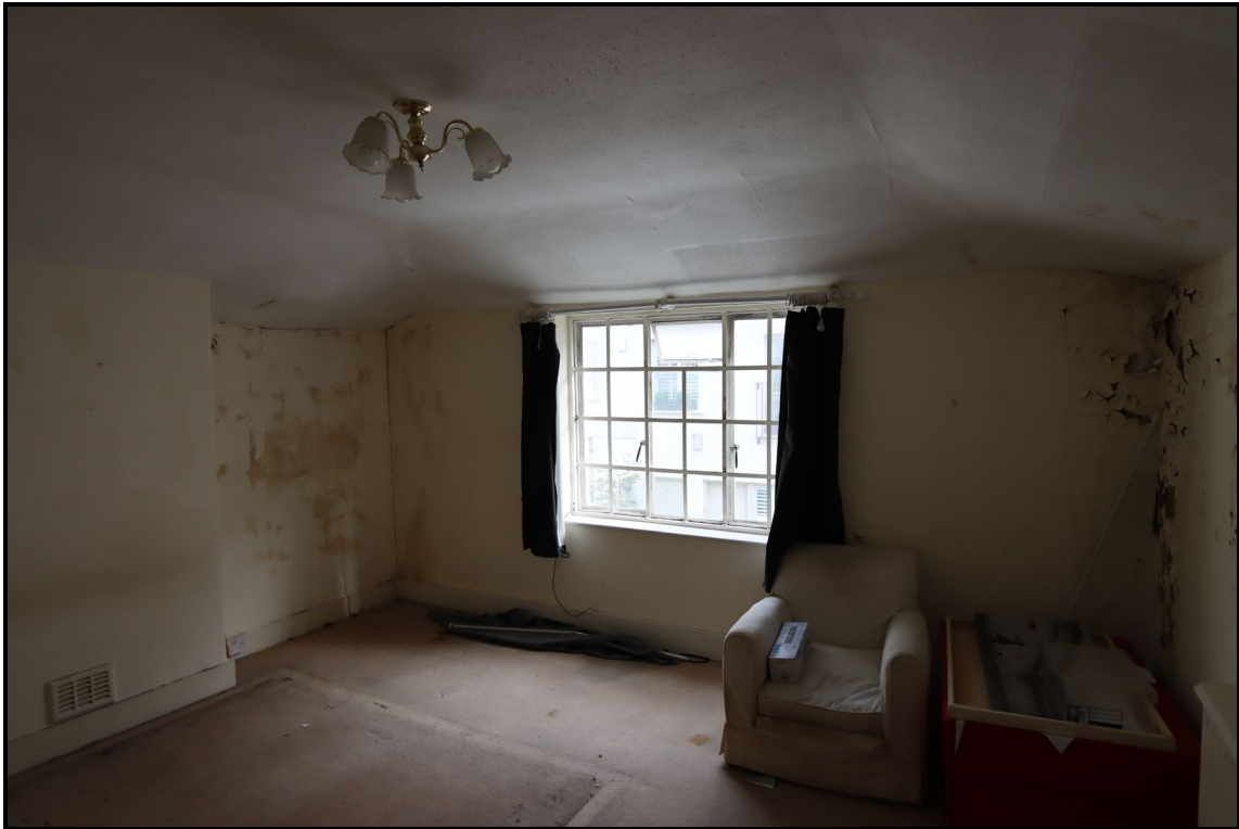
Photo 1 – Front bedroom water damage
