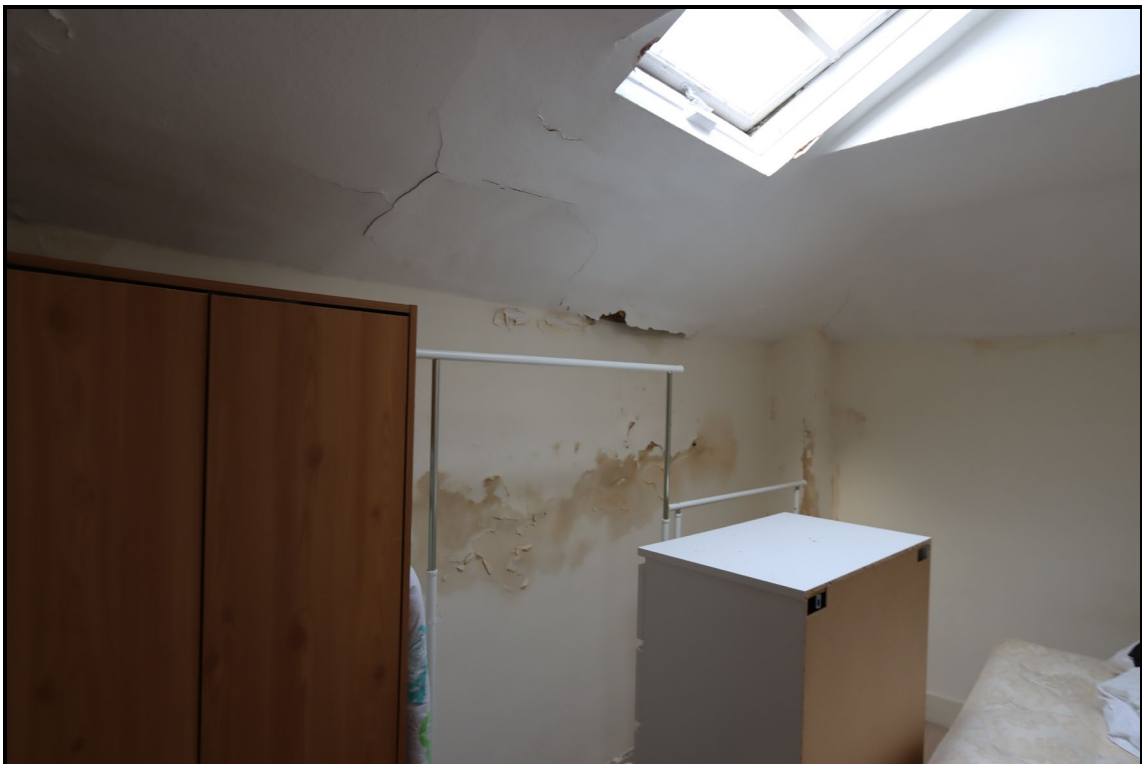
Photo 2 – Rear bedroom water damage
