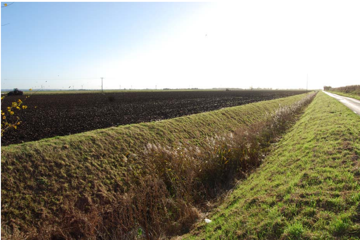
Drain to the west of Quay Lane, view to south.
