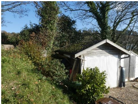
View from Loves Lane looking north east
