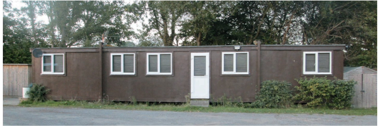
EXISTING PHOTOGRAPH OF THE GATEHOUSE
