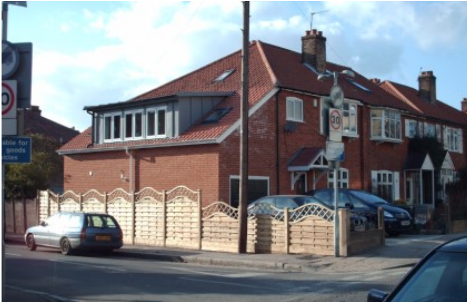
Fig 1. No 136 King Charles Road at junction to King Charles Crescent
