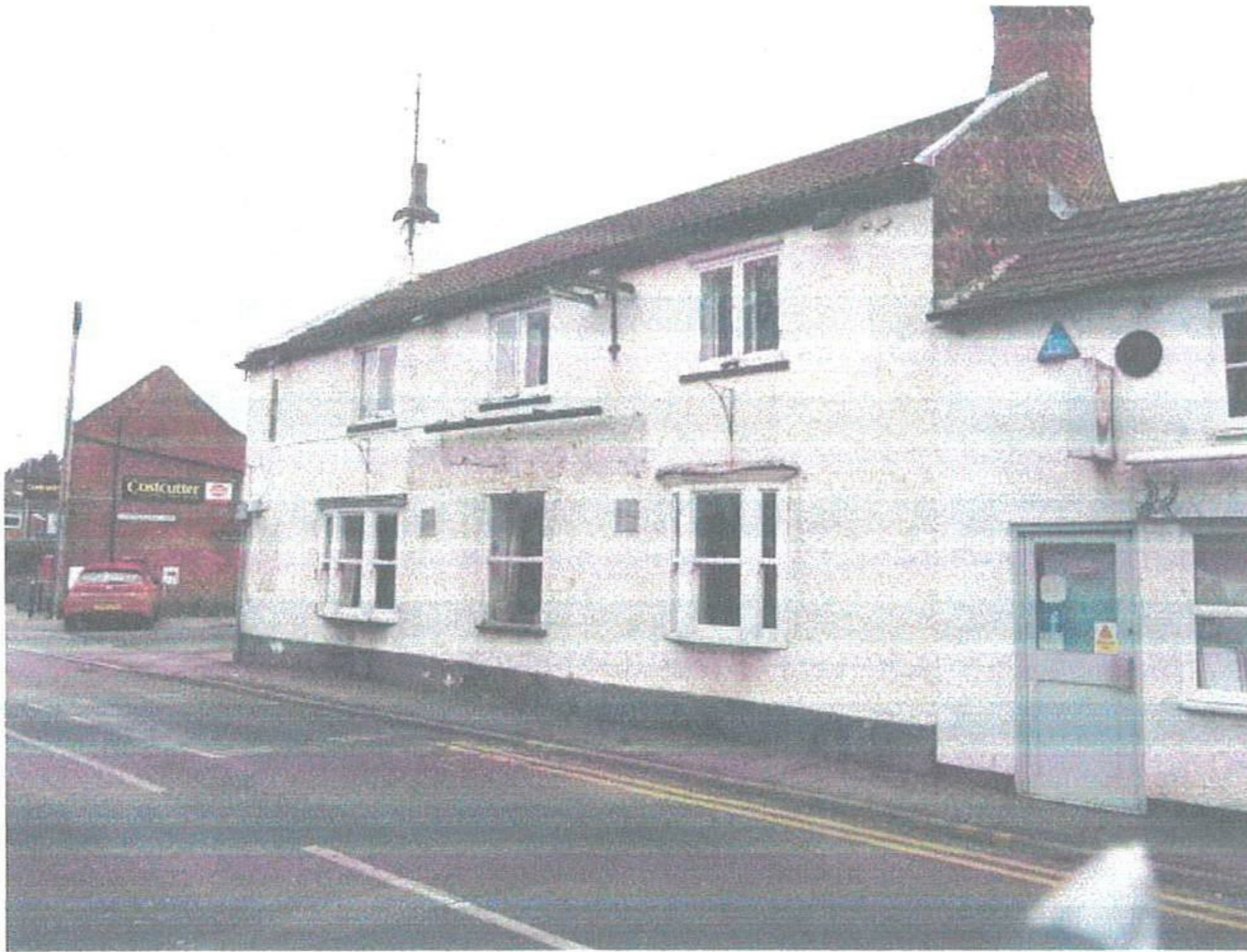
Plate 7. Looking towards the two small outhouses on the north and east elevations.
