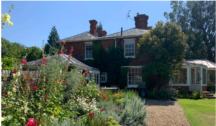
FIG 05 AND 06 - FRONT AND REAR ACCESS TO PROPERTY
