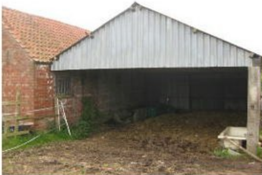
Photograph 3: Exterior of the cattle shelter
