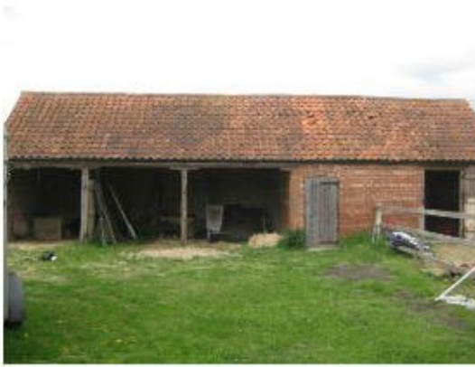
Photograph 1: Exterior view of the barn
