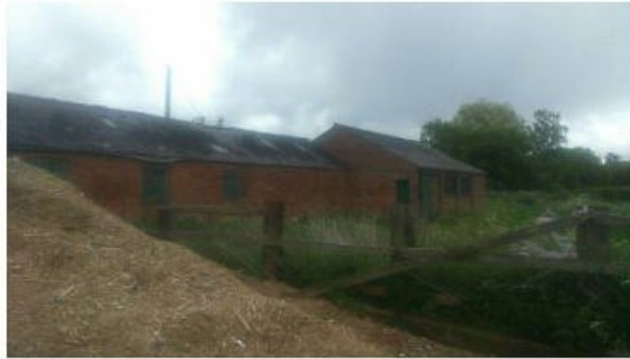
Photograph 4: Western elevation of the L-shaped building
