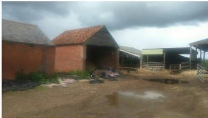
Photograph 2: The detached open-sided building
