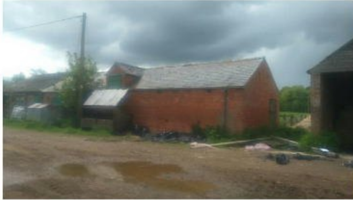
Photograph 1: Eastern elevation of the L-shaped building
