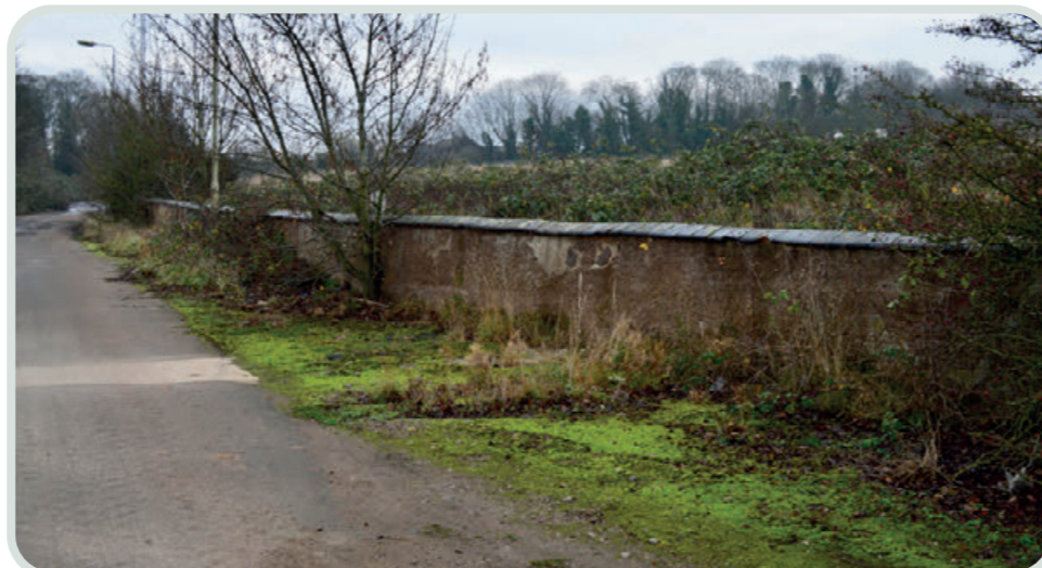
Photo 8: The boundary wall to the landfill site along Harrolds Lane
