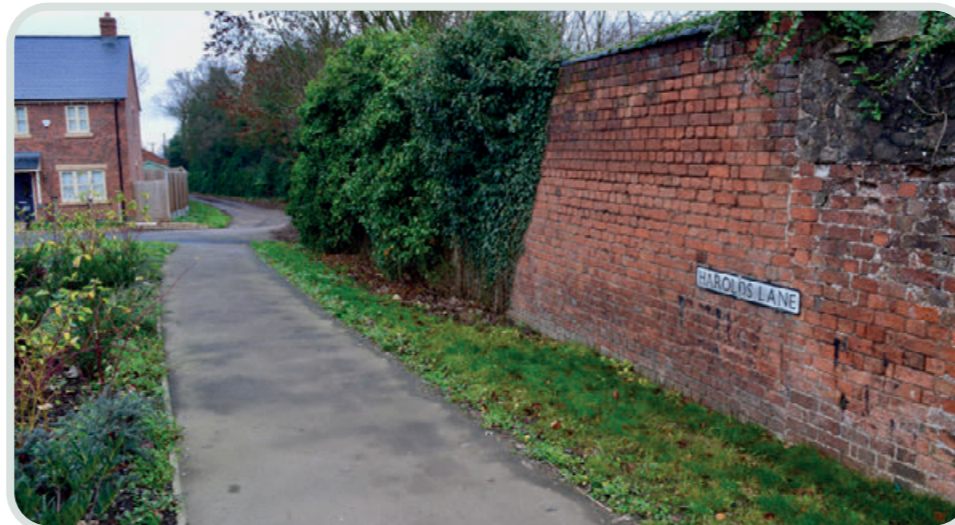
Photo 23: Harrolds Lane at Hall Walk
