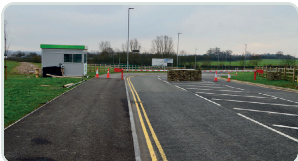
Photo 16: Looking South towards the entrance of SES Phase 1
