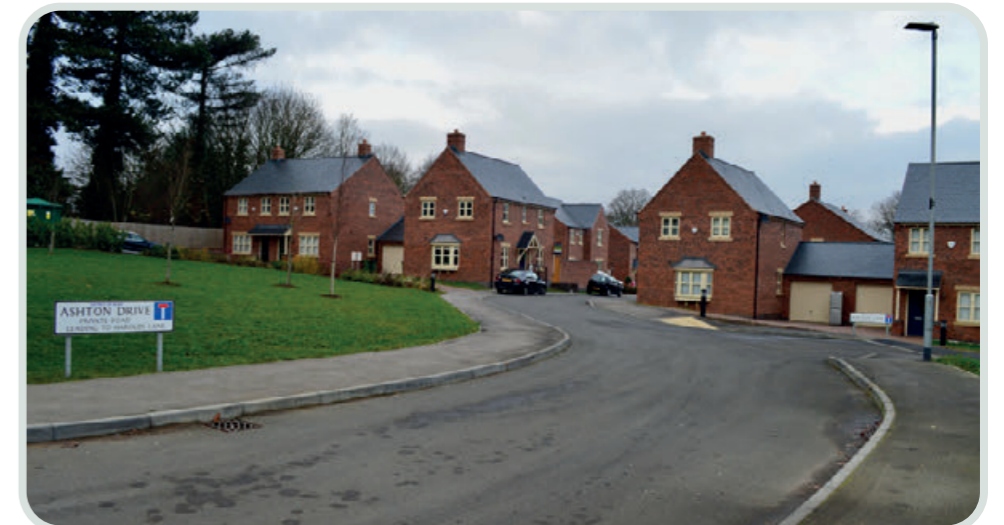
Photo 24: New Homes at Hall Walk
