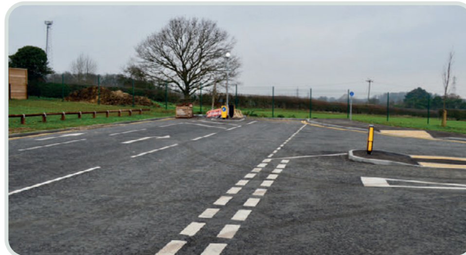
Photo 14: Looking North at the current end of the SES Phase 1
