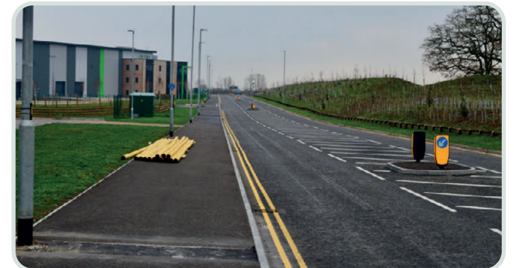
Photo 15: Looking South along the SES Phase 1 Road
