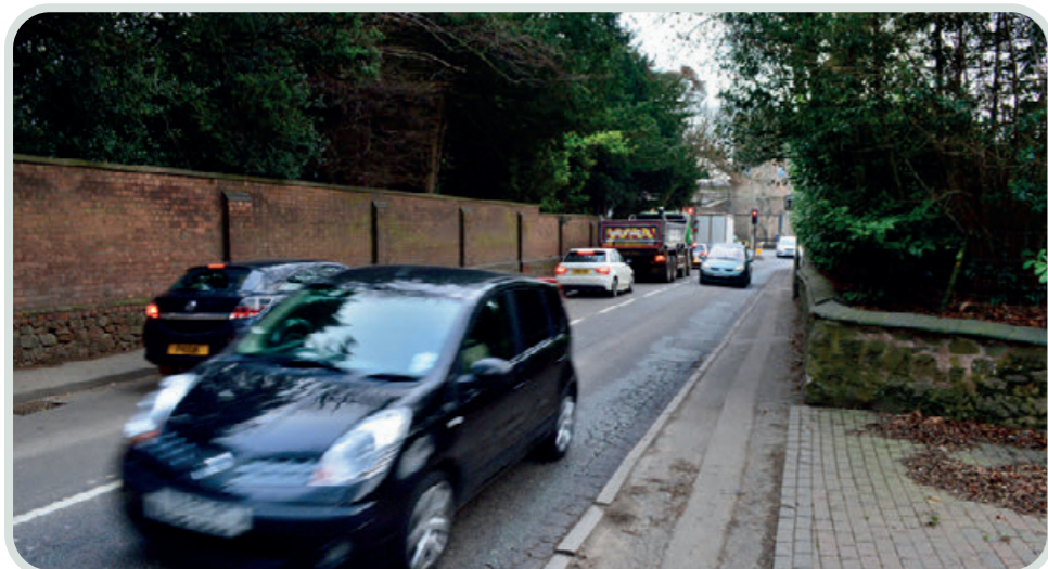
Photo 22: Hall Walk looking South alongside Enderby Hall
