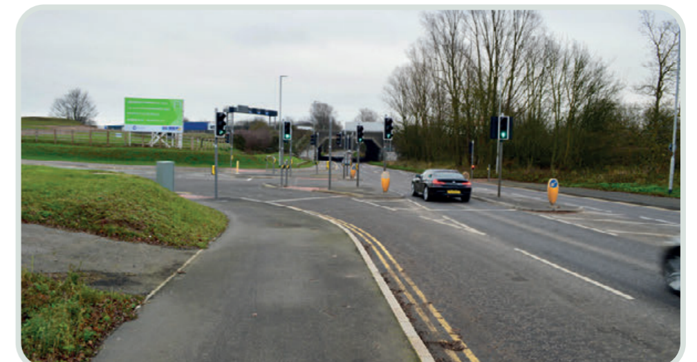
Photo 18: Looking East to the Leicester Lane junction
