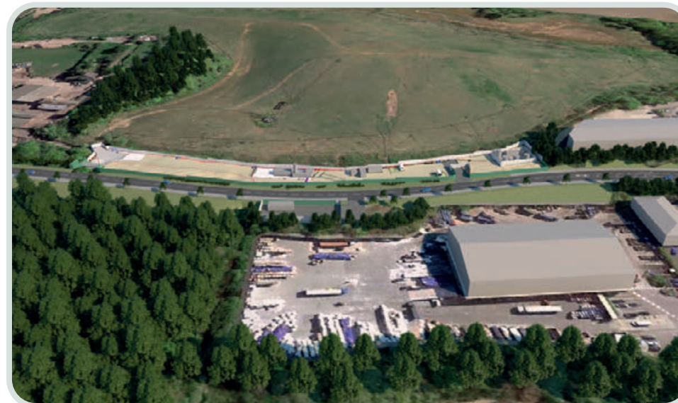
View from the looking towards SUEZ and the landfill site
