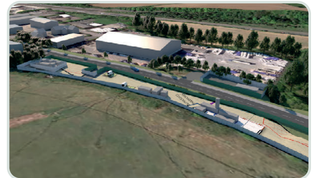
View looking north towards SUEZ compound
