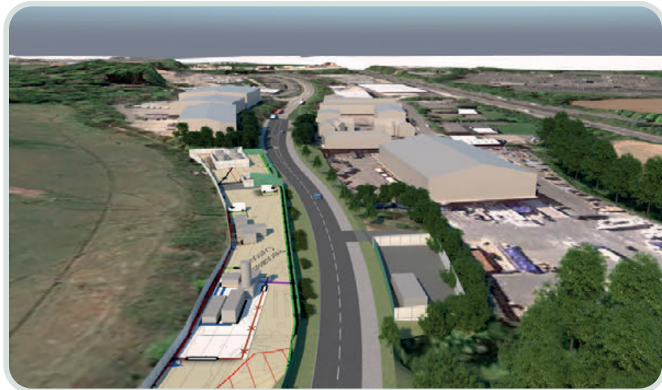
View towards SUEZ and Warrens Industrial estate
