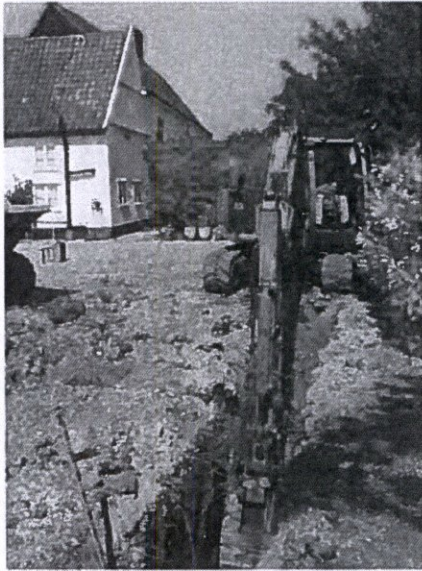
Excavation of footing trench.. Looking west.
