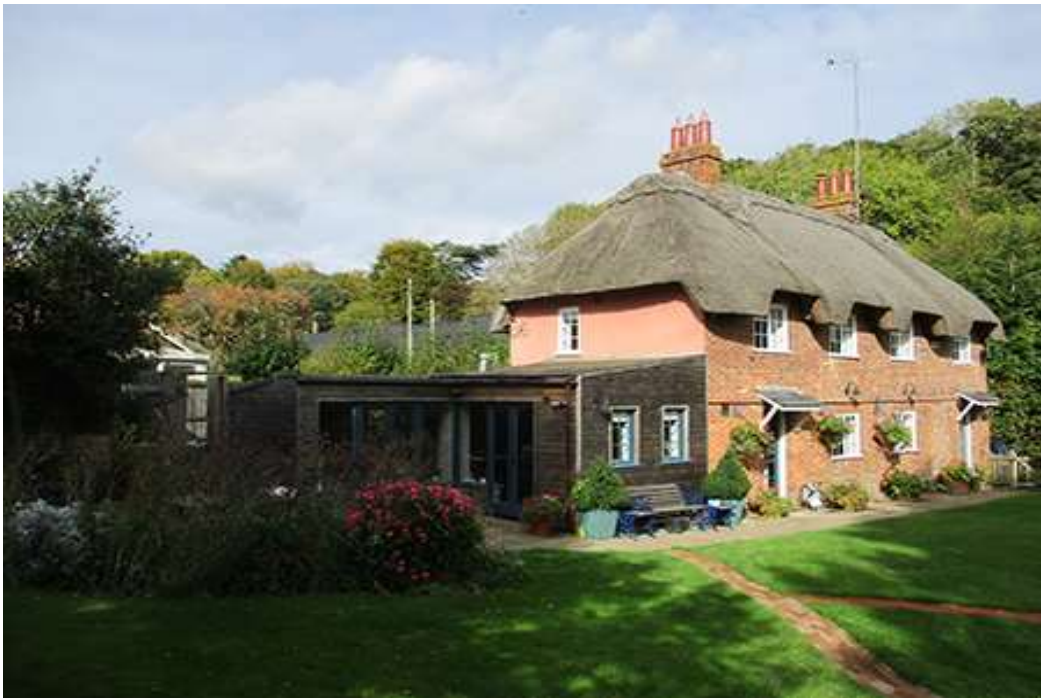
Showing single storey wing/kitchen and area of proposed extension.
