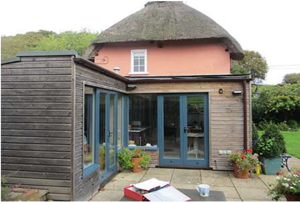
Patio in front of kitchen, area of extension.
